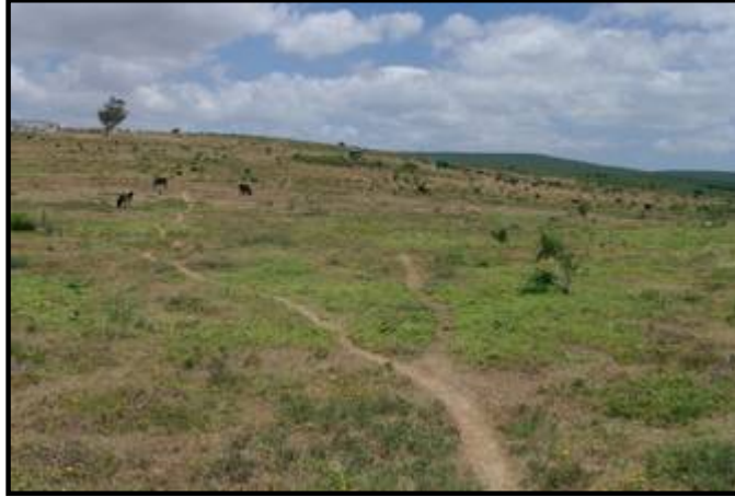
Figure 16: View of the collector sewer alignment route from N8-N9 northwards
