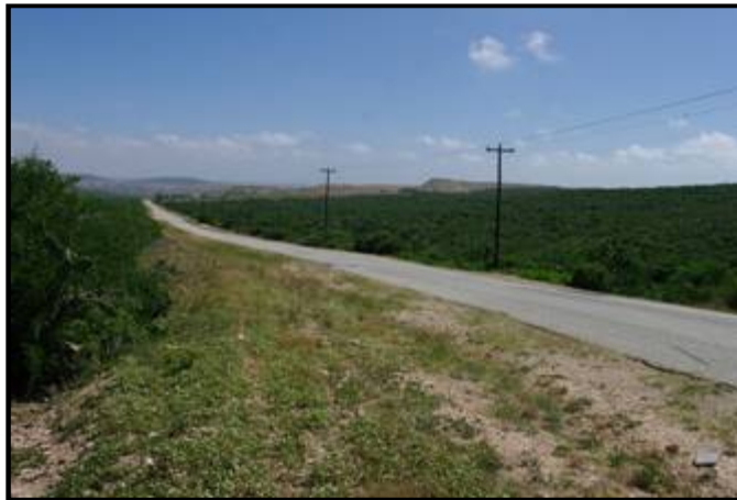
Figure 14: General view of the collector sewer alignment route between N4 and PS1
