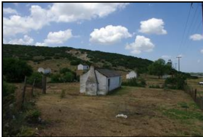
Figure 22: View of the Site BS2 structures from the west
