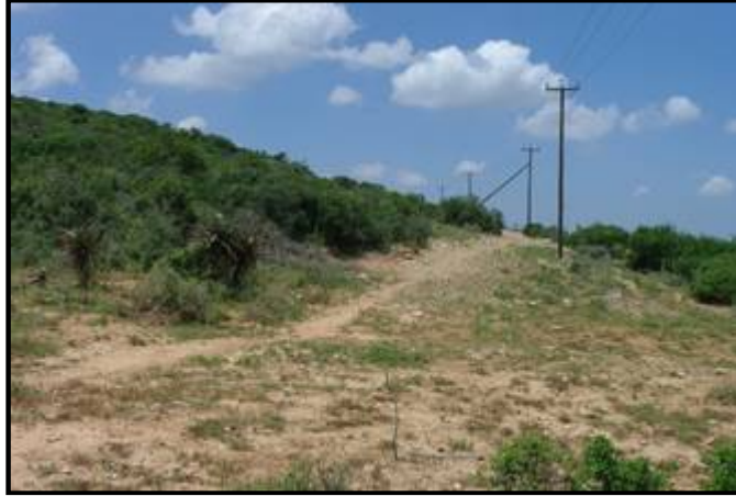
Figure 13: General view of the collector sewer alignment route between PS1 and N35
