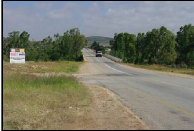
Figure 10: General view of the Option 2 siphon route alignment between N61 and N63
