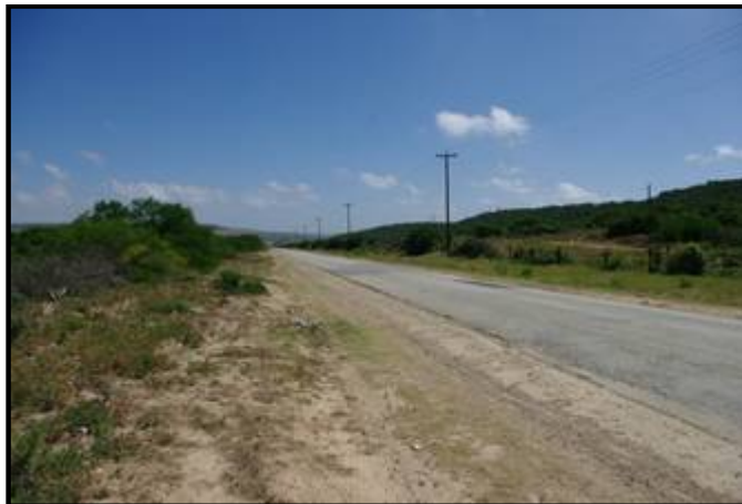
Figure 15: View of the collector sewer alignment route from N6 southwards
