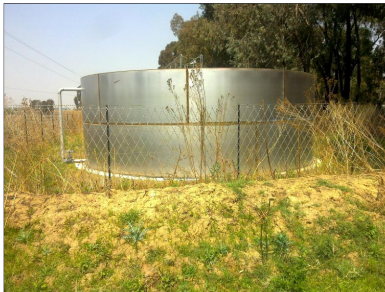
Figure 3: Sewage plant structure at Bantu Bonke.
