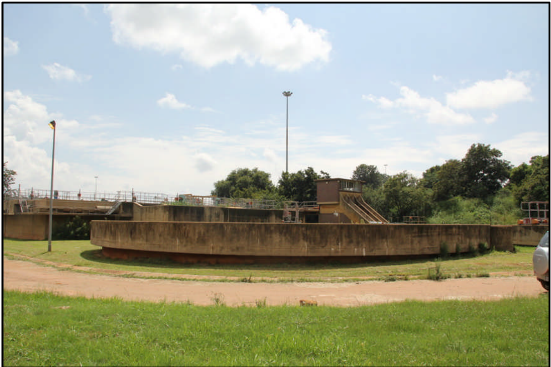
Fig. 5. One of the existing clarifiers on the site.
