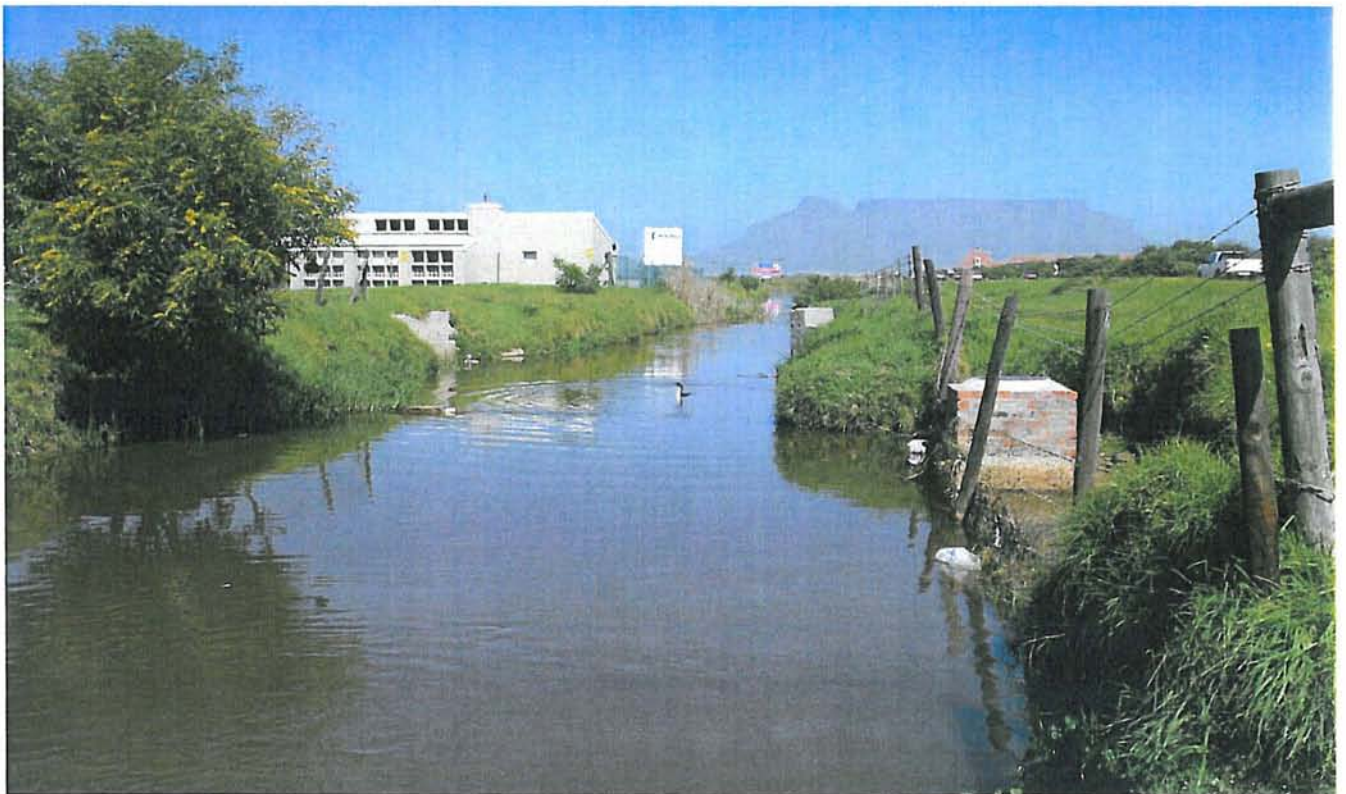
Plate 2 The canal just before it enters Rietvlei. R27 is to the right
