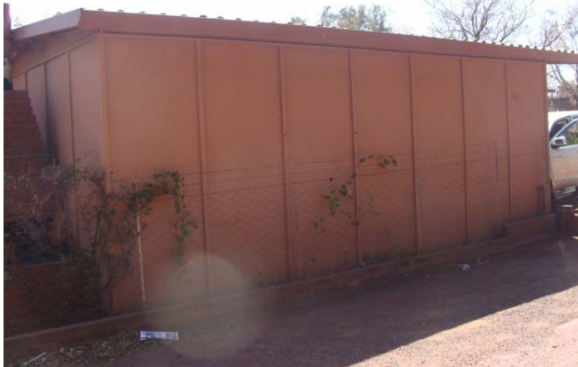
Figure 30 Pre-fabricated garage at one of the houses.
