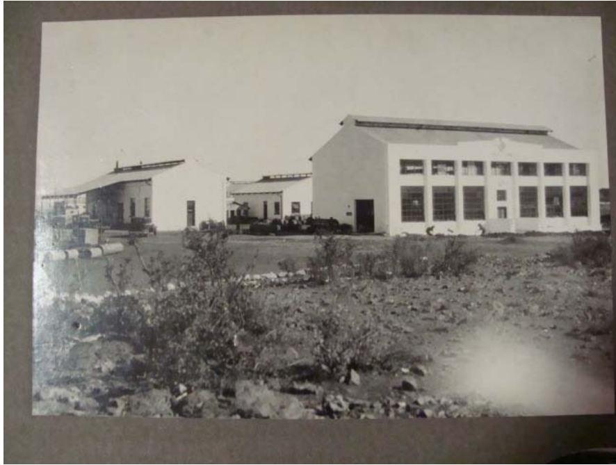
Figure 51 The power station with workshops to its left during the 1930's (ASSMANG Beeshoek collection)
