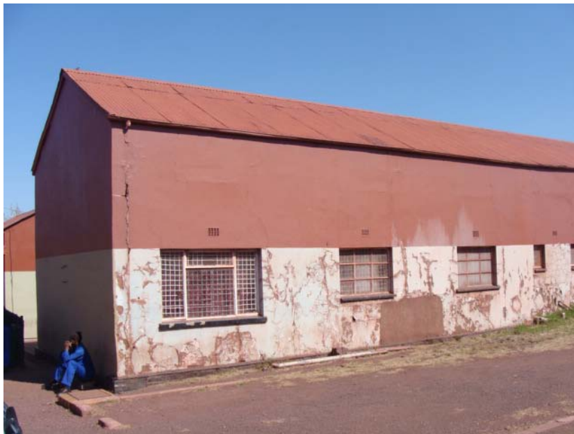
Figure 62 Outside wall of the compound.
