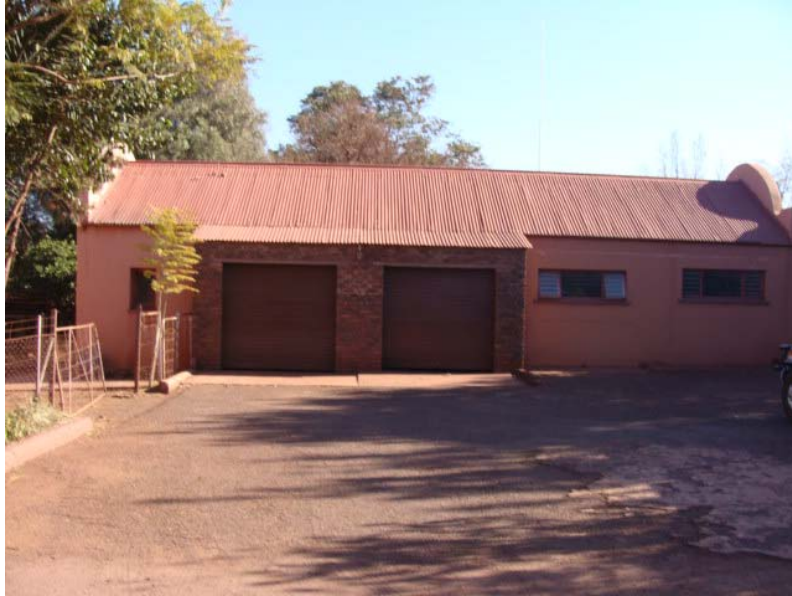
Figure 24 Garages between houses no 12 and 13.
