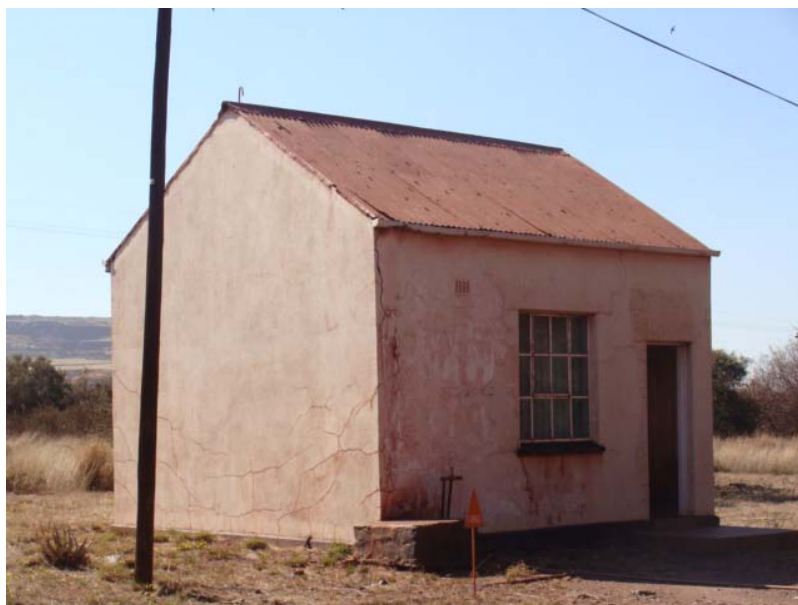
Figure 41 Another, but older, outbuilding behind the technical services building.
