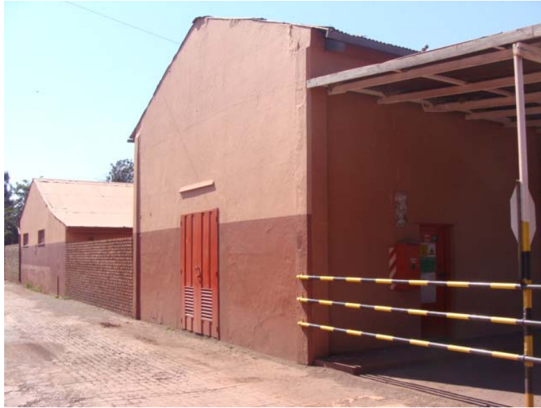
Figure 59 The emergency services buildings.
