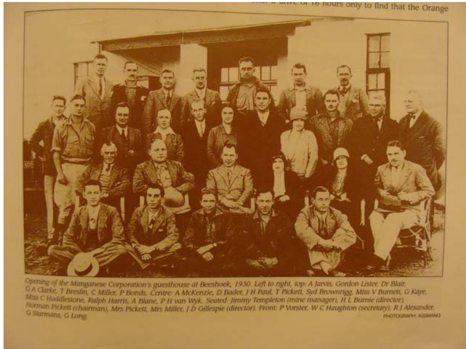
Figure 37 The technical services building when it was opened as a guest house in 1930 (Snyman 2000: 33).
