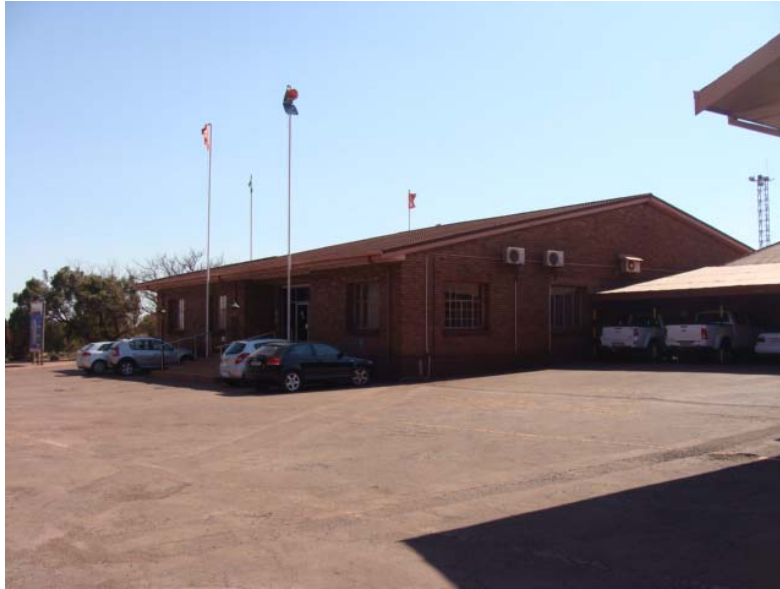
Figure 65 The main office building.
