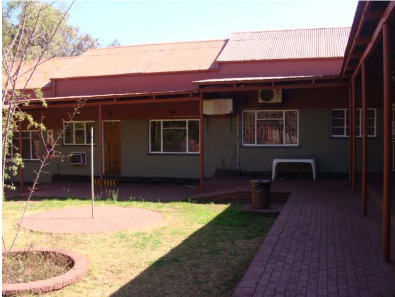
Figure 63 Revamped inside of the compound.
