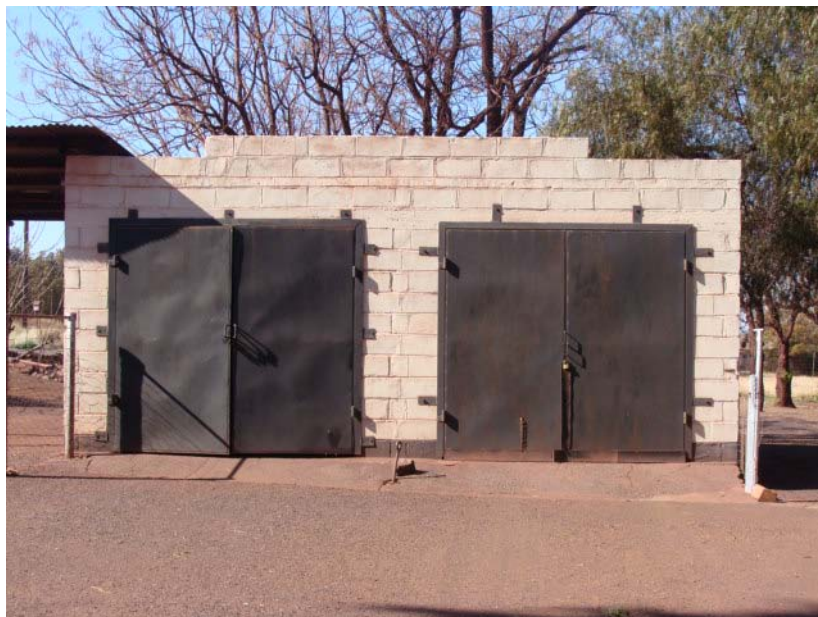
Figure 15 Garages between houses no 5 and 6.
