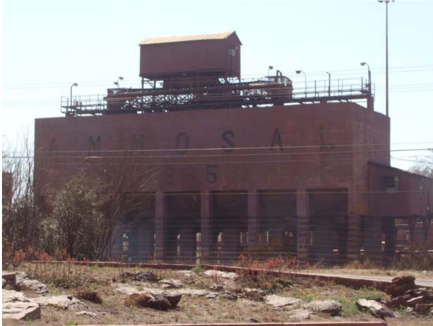
Figure 48 The 1929/30 loading bin.
