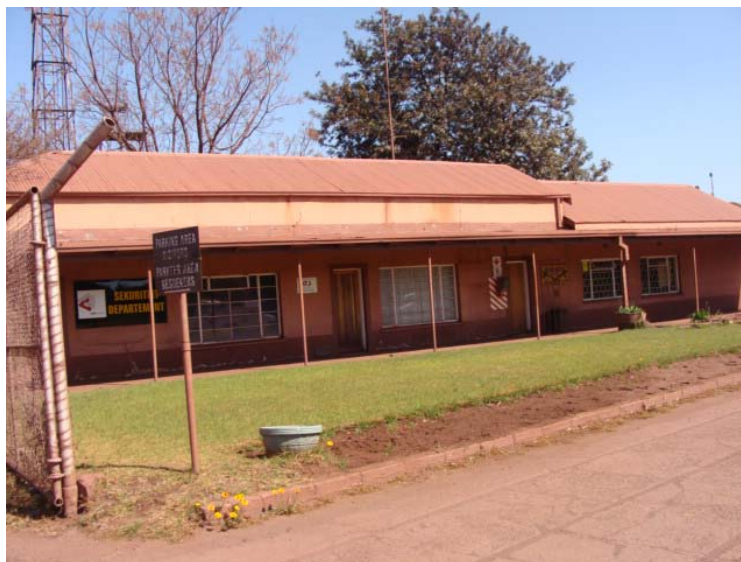
Figure 45 The security building.
