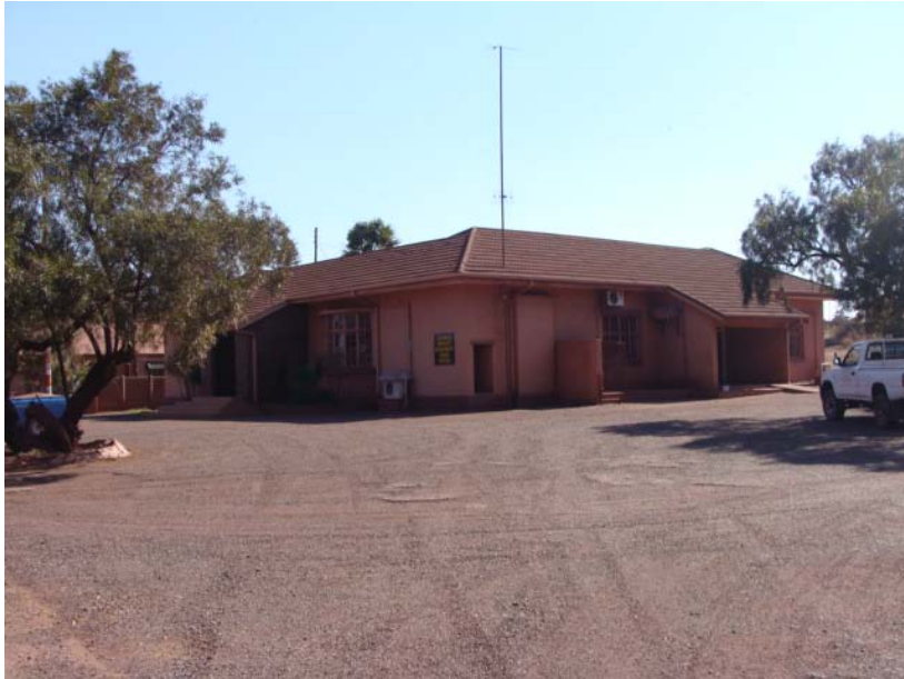
Figure 38 The technical services building.
