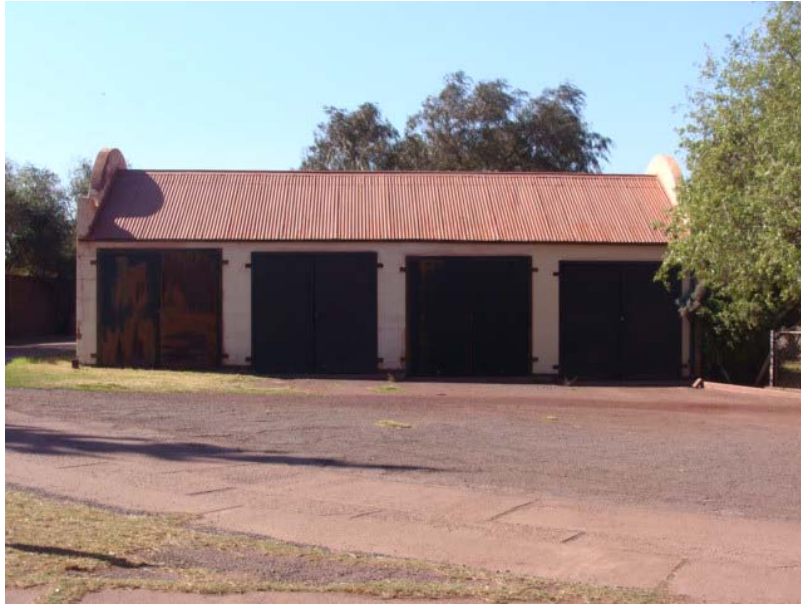
Figure 10 Garages between houses no 1 and 2.
