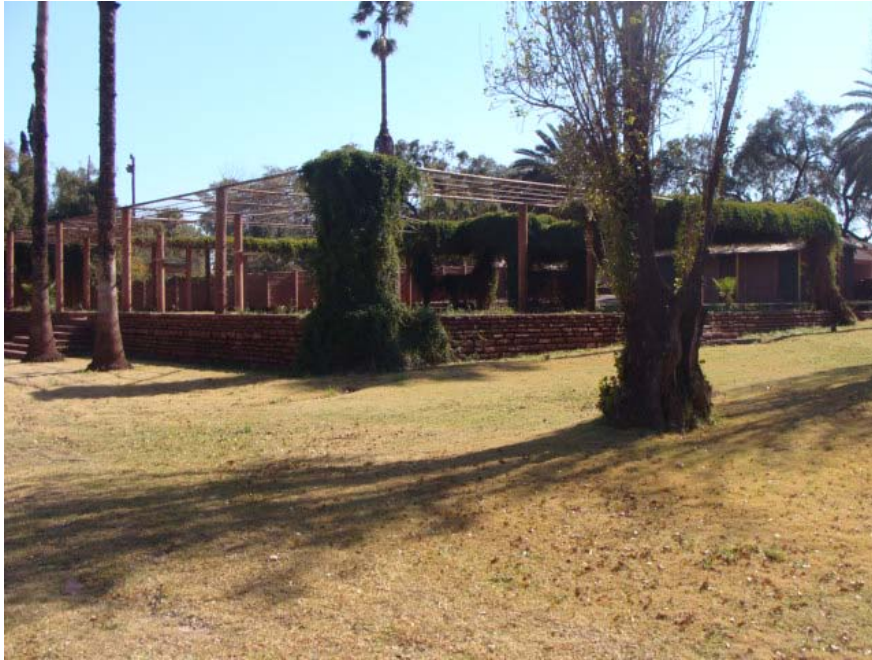
Figure 67 Garden feature in recreation area.
