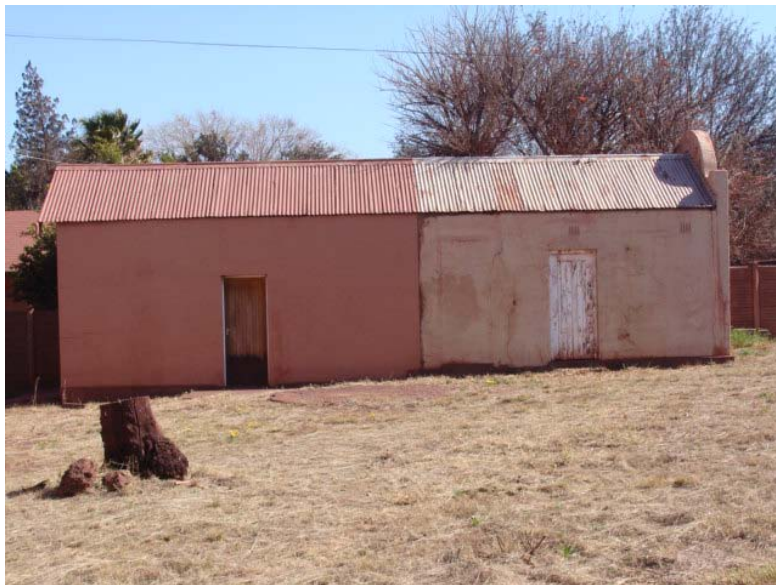
Figure 39 Outbuilding behind the technical services building. Note the later extension on the left hand side.
