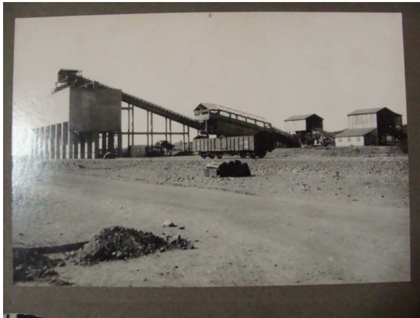
Figure 46 The loading bin dating from 1929/30 (ASSMANG Beeshoek collection).
