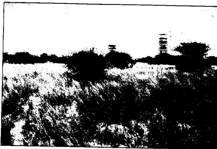
Figure 9: View of the Umtu shaft, currently under construction, from the Umtu Substation development area
