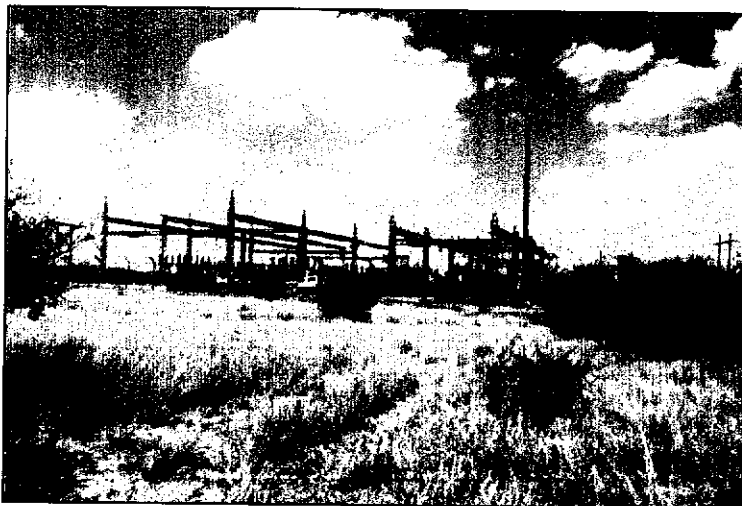
Figure 3: General view of the existing Klipkop Substation
