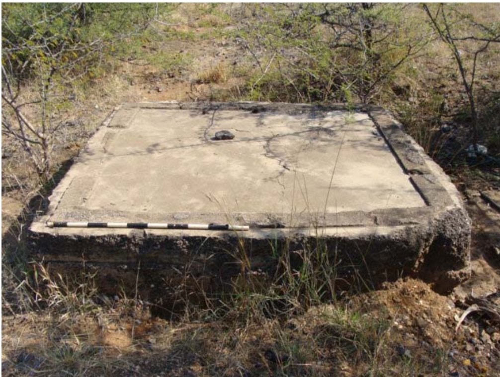
Figure 9 Concrete platform such as this one are found at site no. 2.
