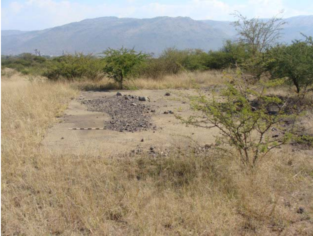
Figure 10 A concrete floor such as some of those at site no. 2.
