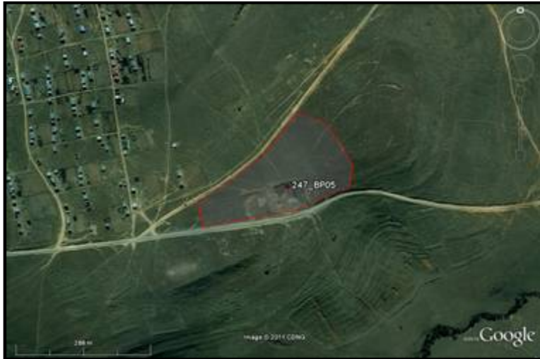
Figure 131: Borrow pit 247_BP05
