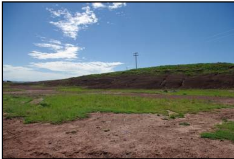
Figure 195: View of borrow pit 042_BP05
