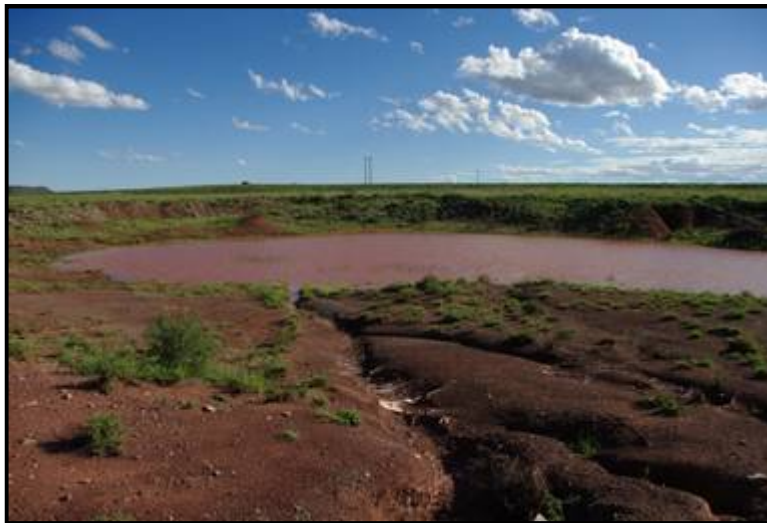
Figure 73: View of borrow pit 660_BP04
