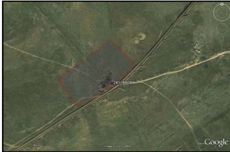
Figure 179: Borrow Pit 261_BP09
