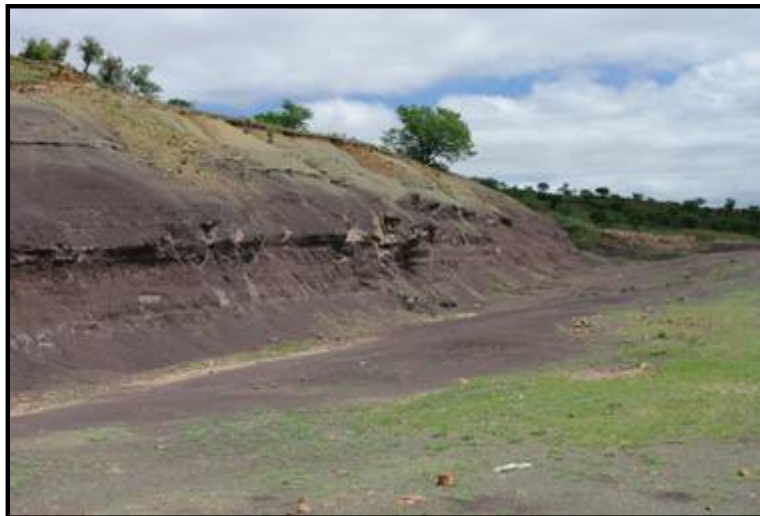
Figure 29: View of borrow pit 732_BP05
