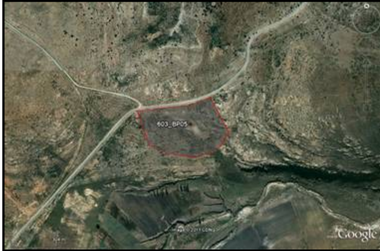
Figure 87: Borrow Pit 603_BP05
