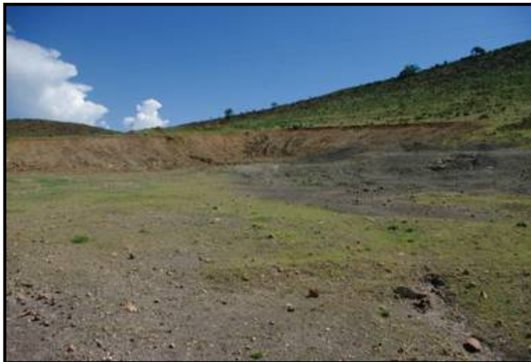
Figure 95: General view of borrow pit 567_BP03
