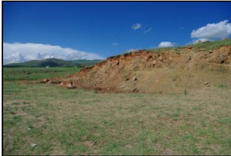
Figure 154: View of the northern portion of borrow pit 038_BP03
