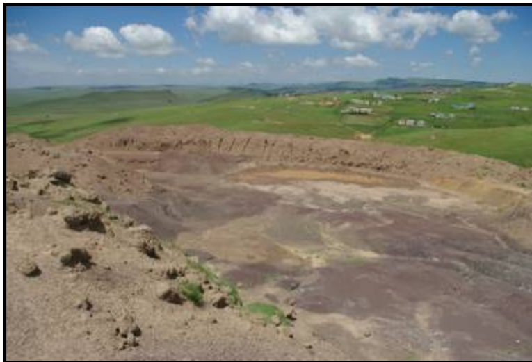
Figure 106: View of a portion of borrow pit 050_BP02
