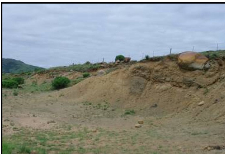
Figure 22: An exposed section of borrow pit 732_BP02
