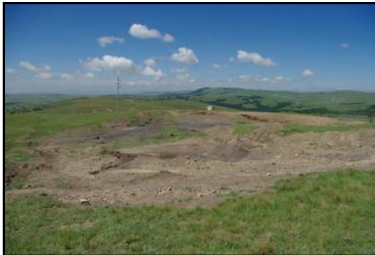
Figure 126: View of borrow pit 247_BP02
