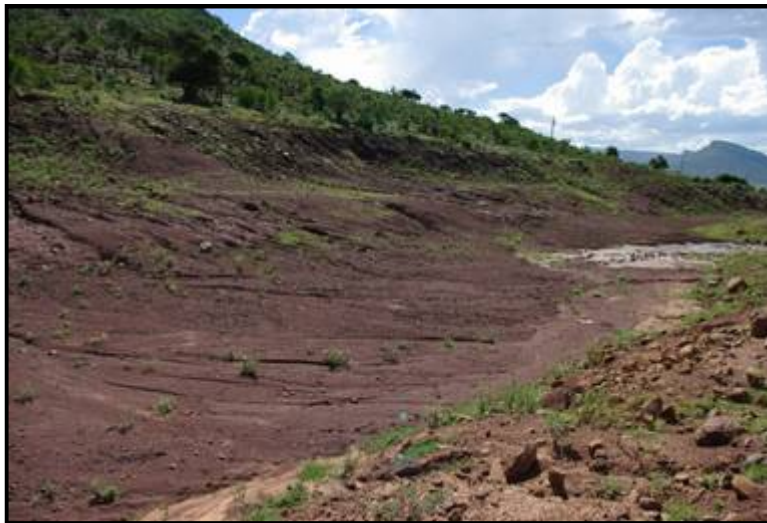
Figure 101: View of a portion of borrow pit 567_BP07
