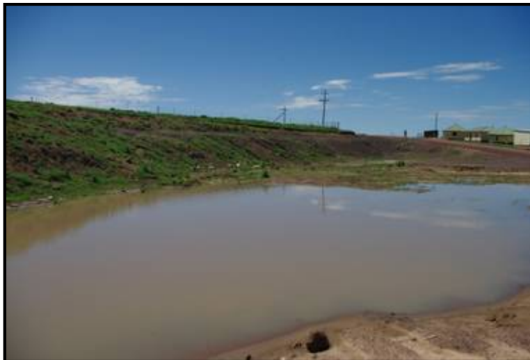
Figure 208: View of borrow pit 381_BP02
