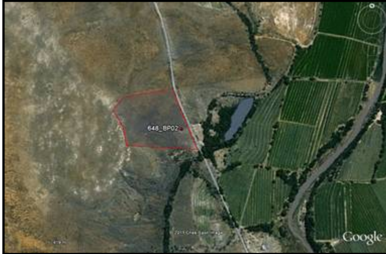
Figure 59: Borrow Pit 648_BP02
