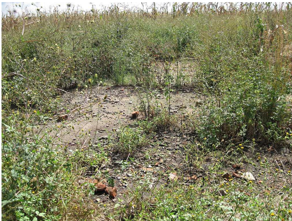
Figure 11. Site BP 4 The remains of an old circular cement dam
