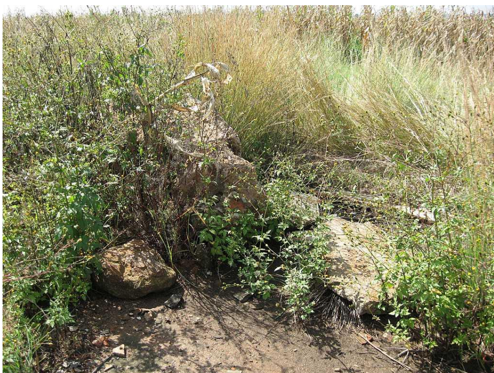
Figure 12. Site BP 4 The remains of an old circular cement dam
