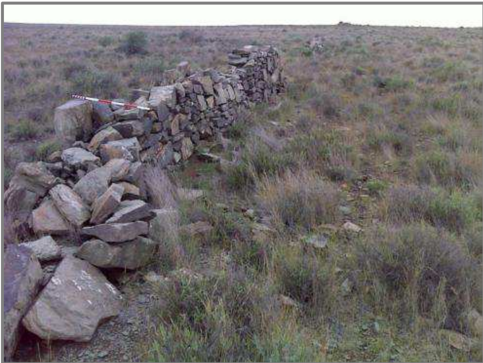
Figure 24. View of the dry packed stone wall.
