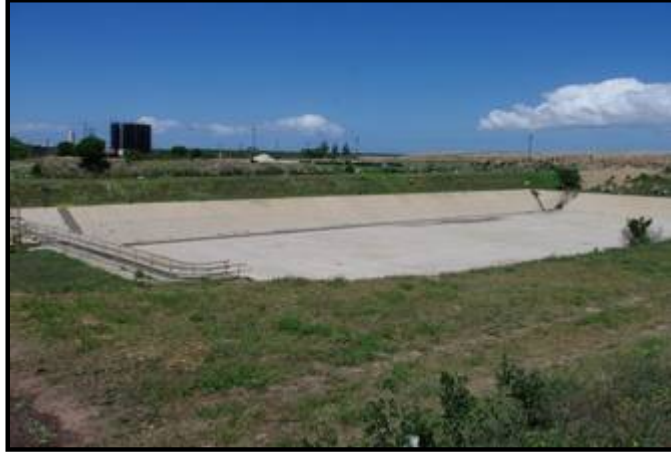
Figure 5: Existing development on the south-eastern portion of the proposed Brickfields pre-treatment works study site - 1
