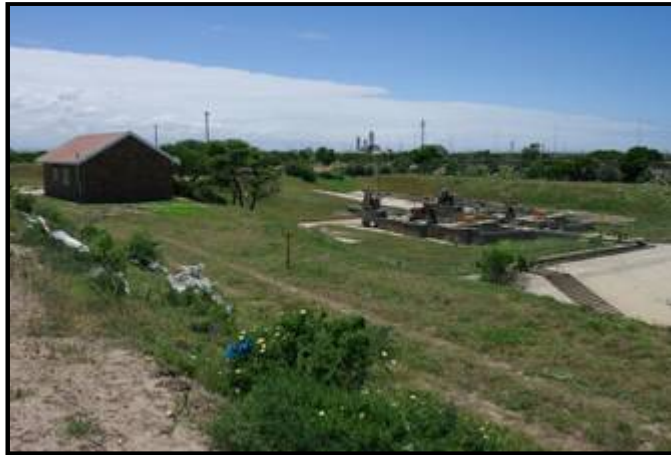
Figure 6: Existing development on the south-eastern portion of the proposed Brickfields pre-treatment works study site - 1
