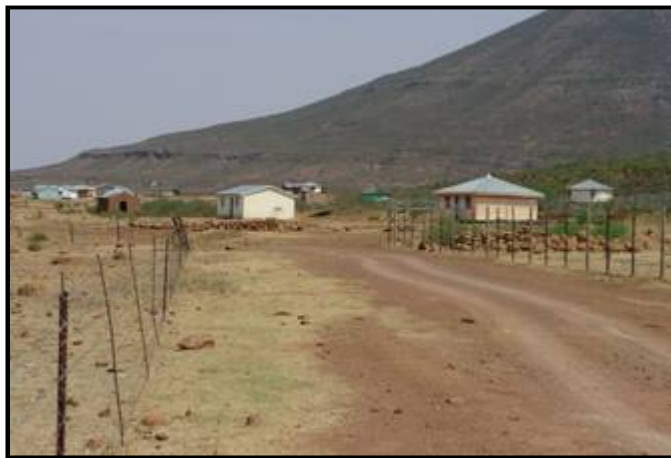
Figure 64: Fairly well defined road reserves at portions of Damane-Mtyintyini
