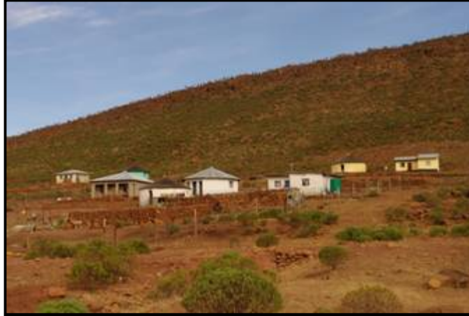
Figure 97: Stone, remaining an important building medium (Kabisweni Village)
