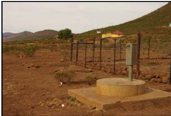
Figure 96: Existing water infrastructure at Kabisweni Village
