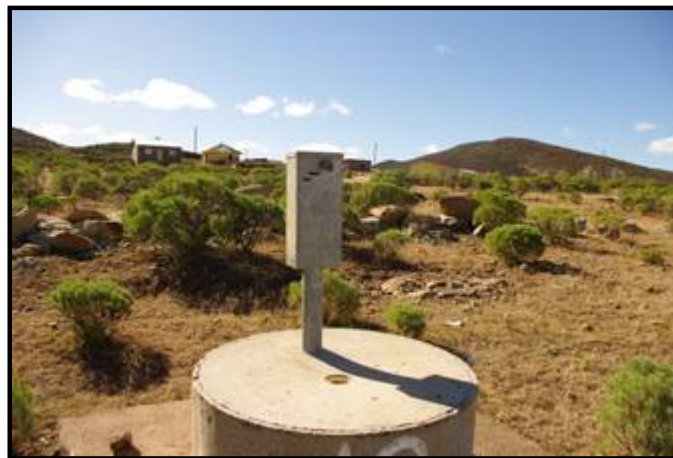
Figure 14: Existing water related infrastructure with a view of the village in the background
