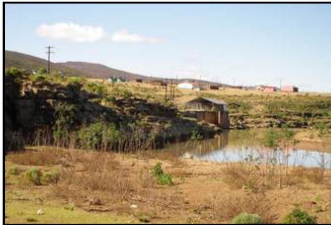
Figure 19: View of the existing pump station
