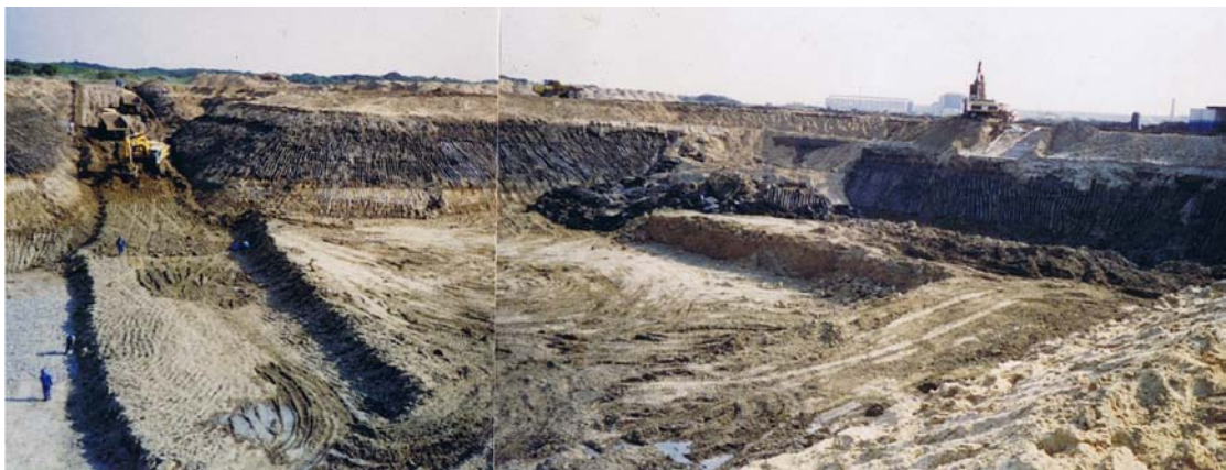
Excavations of dry pit as on 29 July 2005.
