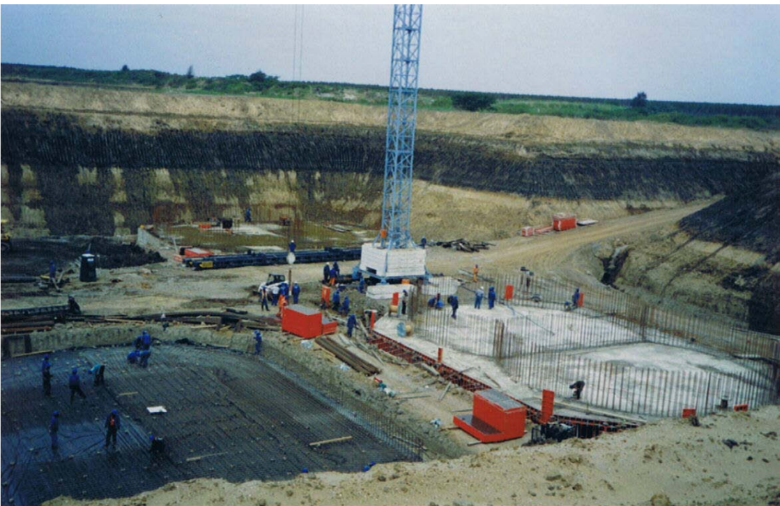
Caissons under construction.
