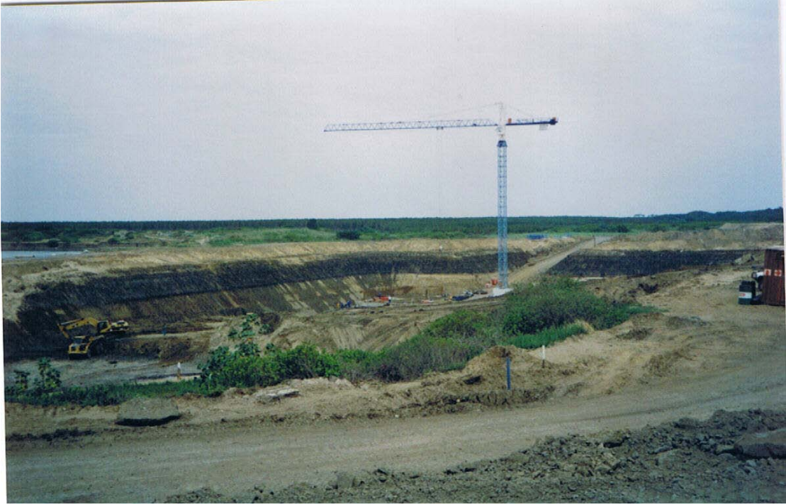
Crane erected in dry pit for construction of first caisson, 16 September 2005.
