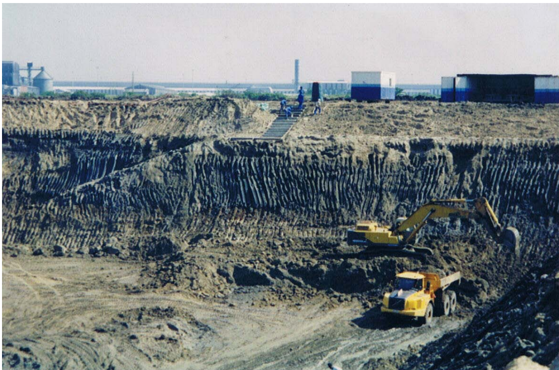
Excavations in progress, 2 August 2005.
