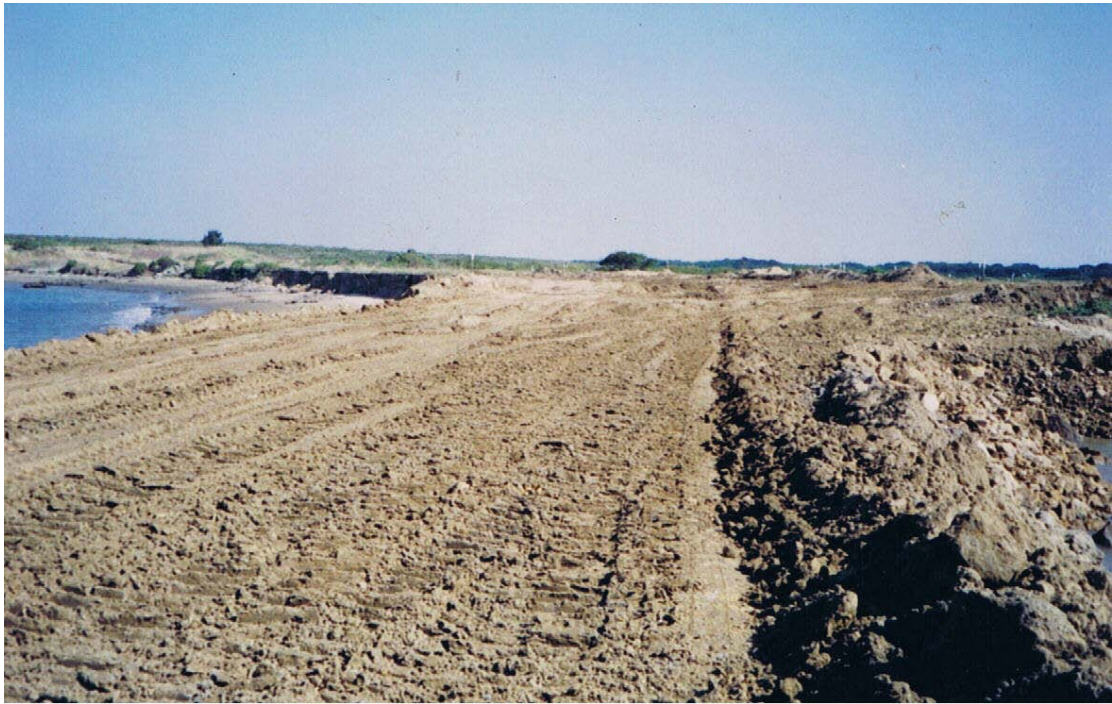
“Wall” between harbour and dry pit excavations.
