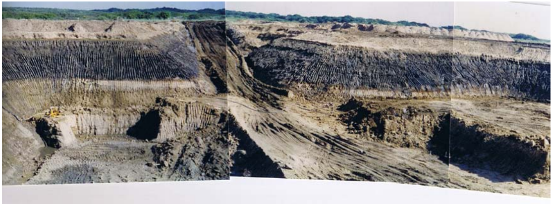
Excavations of dry pit as on 29 July 2005.
