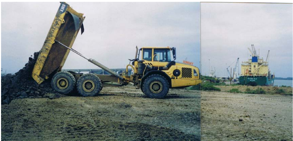
Dumping material from cretaceous layer, 16 September 2005.
