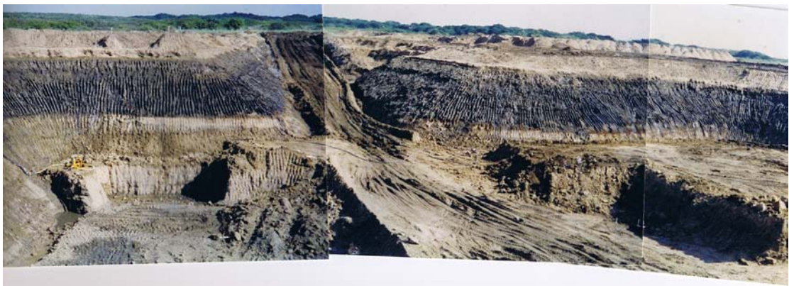
Excavations of dry pit as on 29 July 2005.
