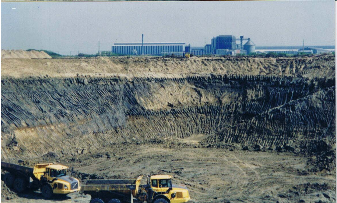
Excavations in progress, 2 August 2005.
