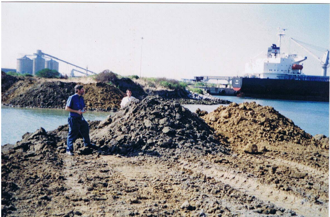
Construction of "wall" between harbour and dry pit excavations, 29 July 2005.
