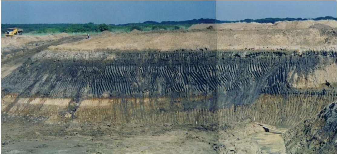
Southern wall of excavation pit, 16 August 2005.
