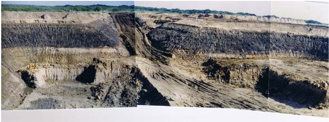
Excavations of dry pit as on 29 July 2005.
