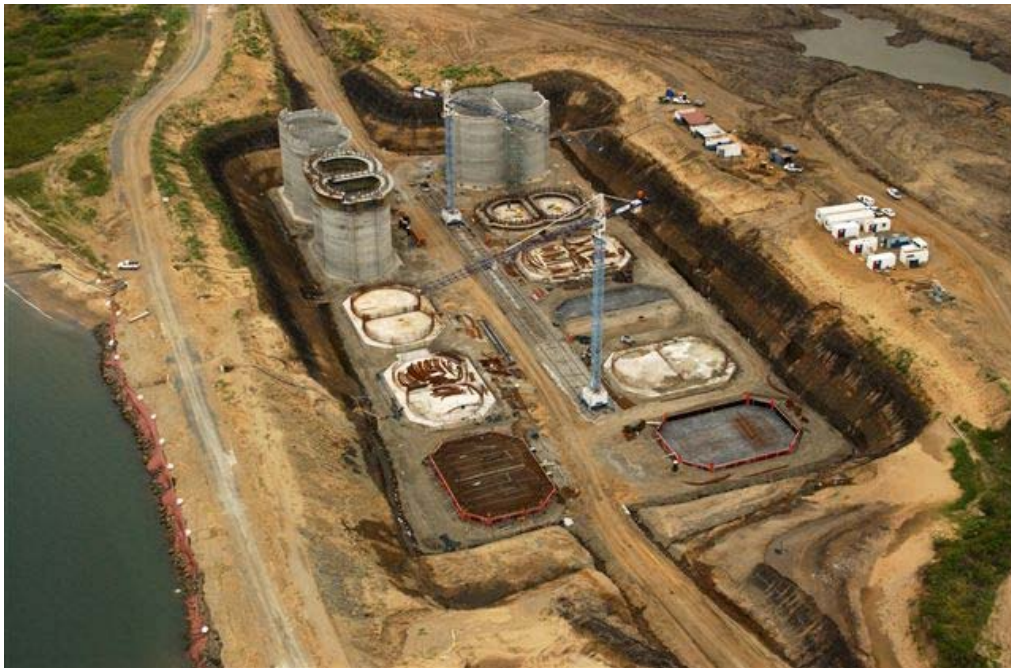
Berm Wall and caissons under construction
