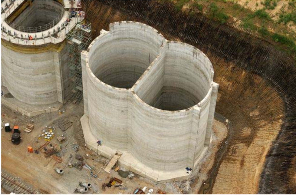
Close up picture of caisson.
