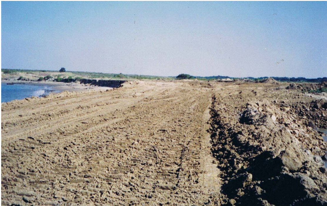
“Wall” between harbour and dry pit excavations.
