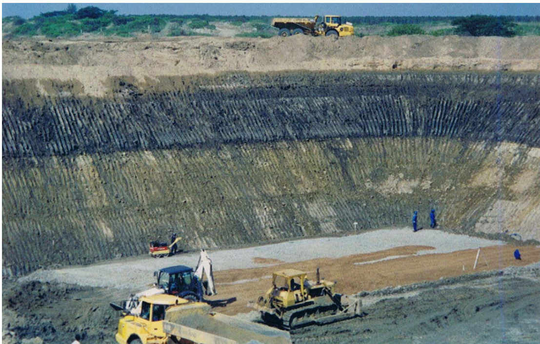
Mechanical excavator, front-end loader and dump truck excavation pit, 2 August 2005.
