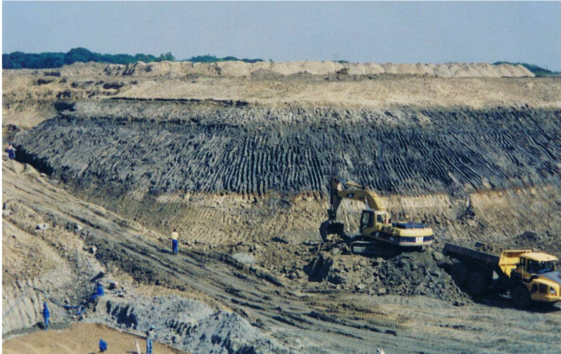
Excavations in progress, 2 August 2005.
