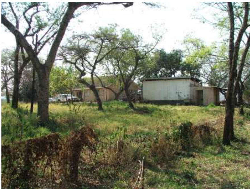
Fig. 5. Site 4. Site NC 4. A house just outside the proposed development area.
