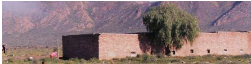
Fig. 5. The brick 'smoke house' the only standing structure, due for demolition
