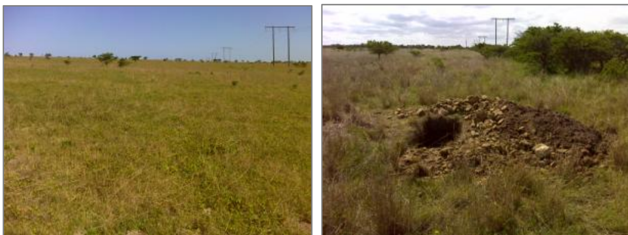
Figs 24-25. Examples of disturbances such as Eskom power lines and the newly dug holes.
