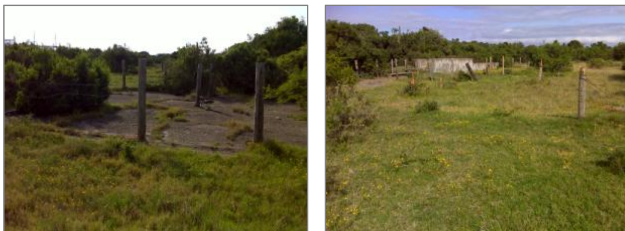
Figs 30-31. Views of the paving and dipping tank at the area marked CS-B1.
