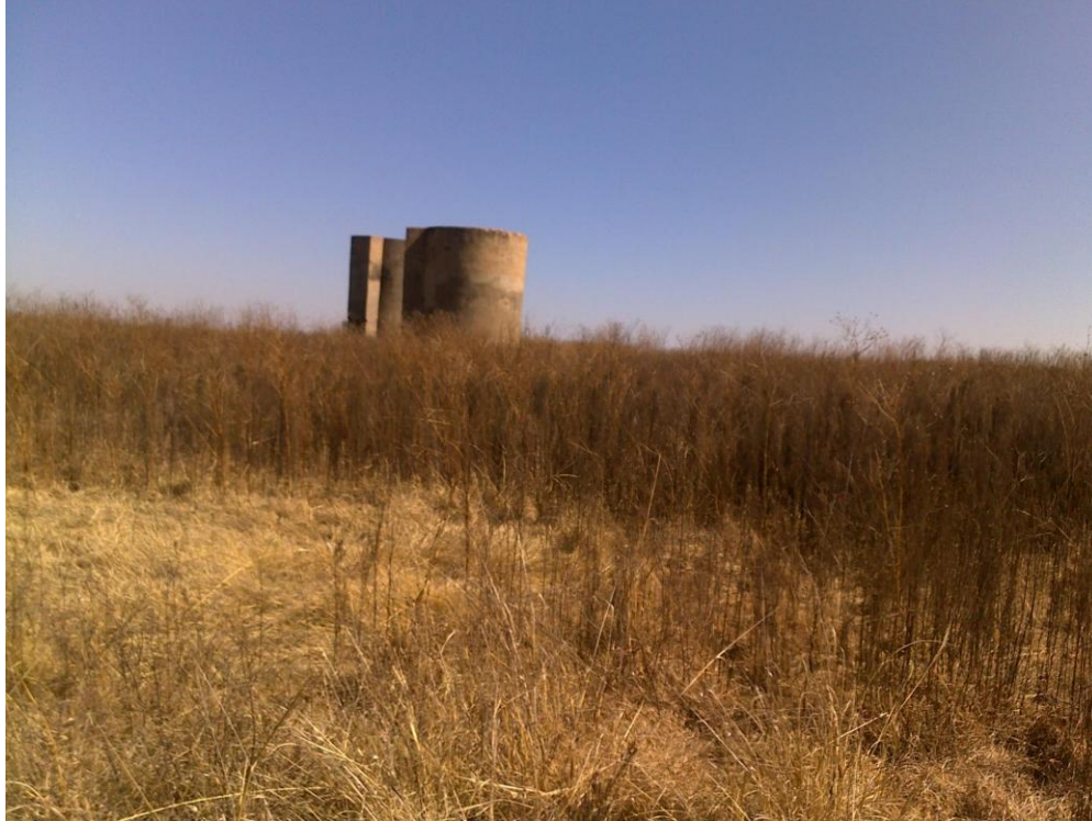
Figure 4: View of the old Silos within the proposed site.
