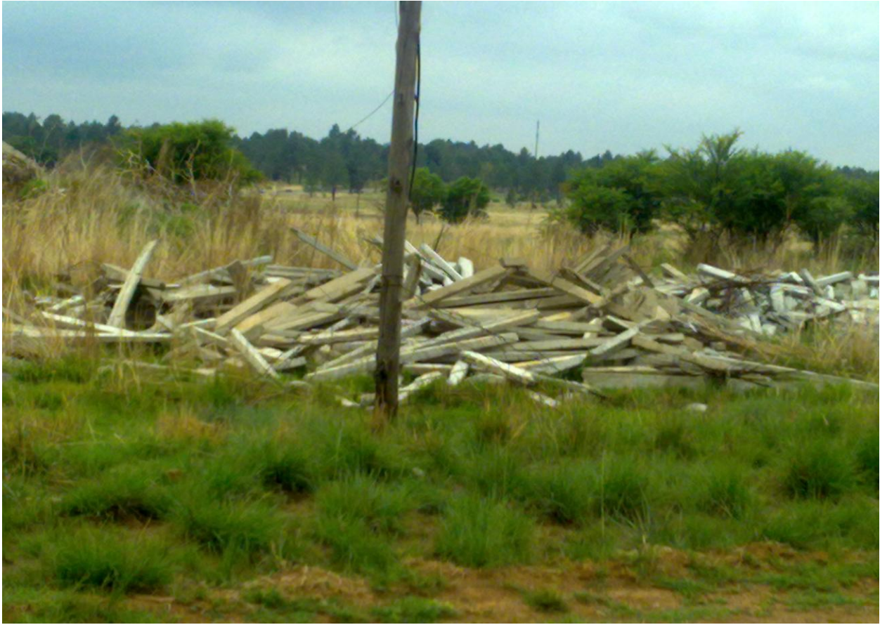
Picture 1: Durawall panels on site
