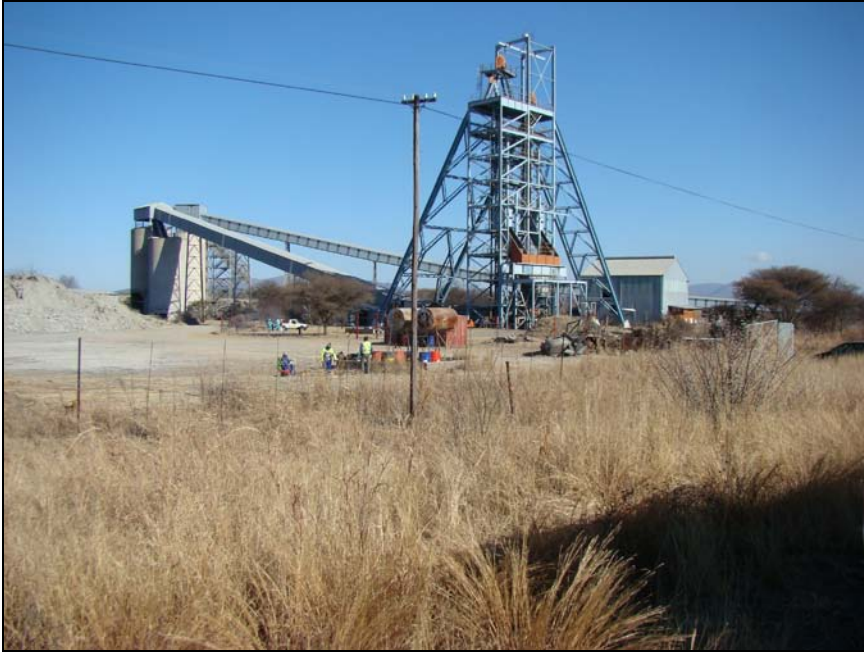
Fig.36 Existing mine at Point A, Schilpadnest 385KQ, Northam.
