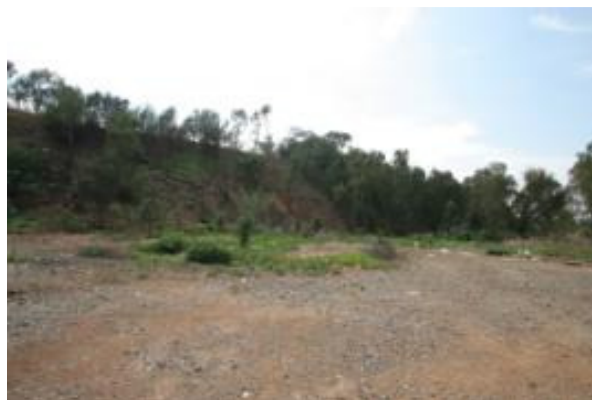
Figure 1: South-eastern view of Slimes Dam 3/L/42
