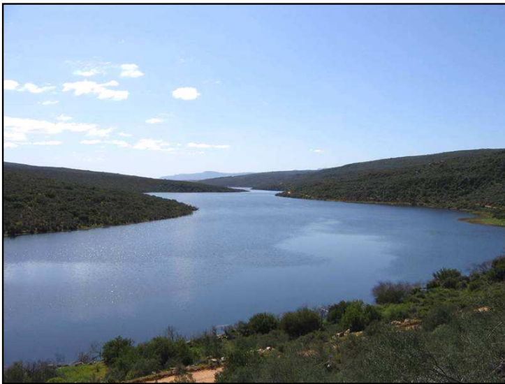
Plate 1: View over part of The Clanwilliam Dam showing the inundated Oliphants River Valley.
