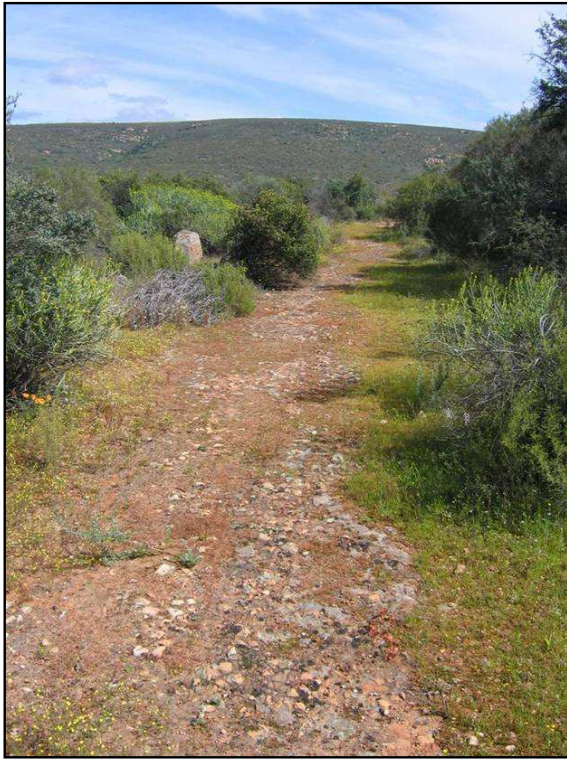
Plate 28: CDE56. A section of the 1860 road with the surface remaining intact. It appears to be of compacted gravel and fossil termiterium.
