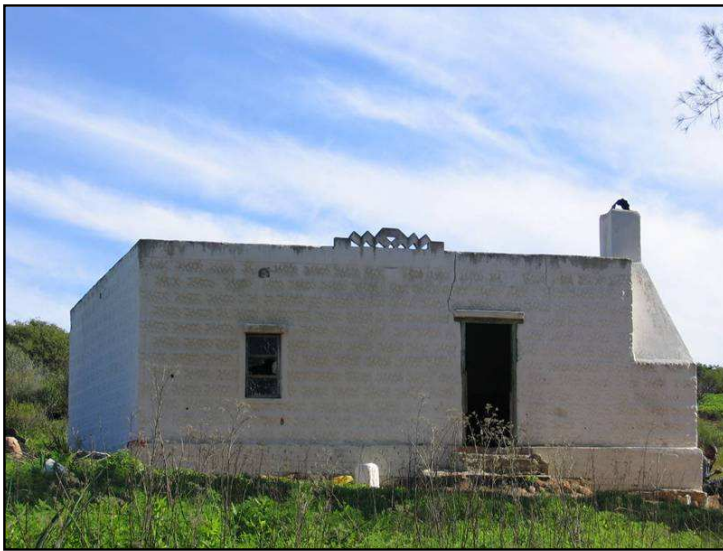
Plate 23: CDW27. An example of an historic structure that is still currently in use as a residence. This cottage probably dates to about the 1930's or 1940's.
