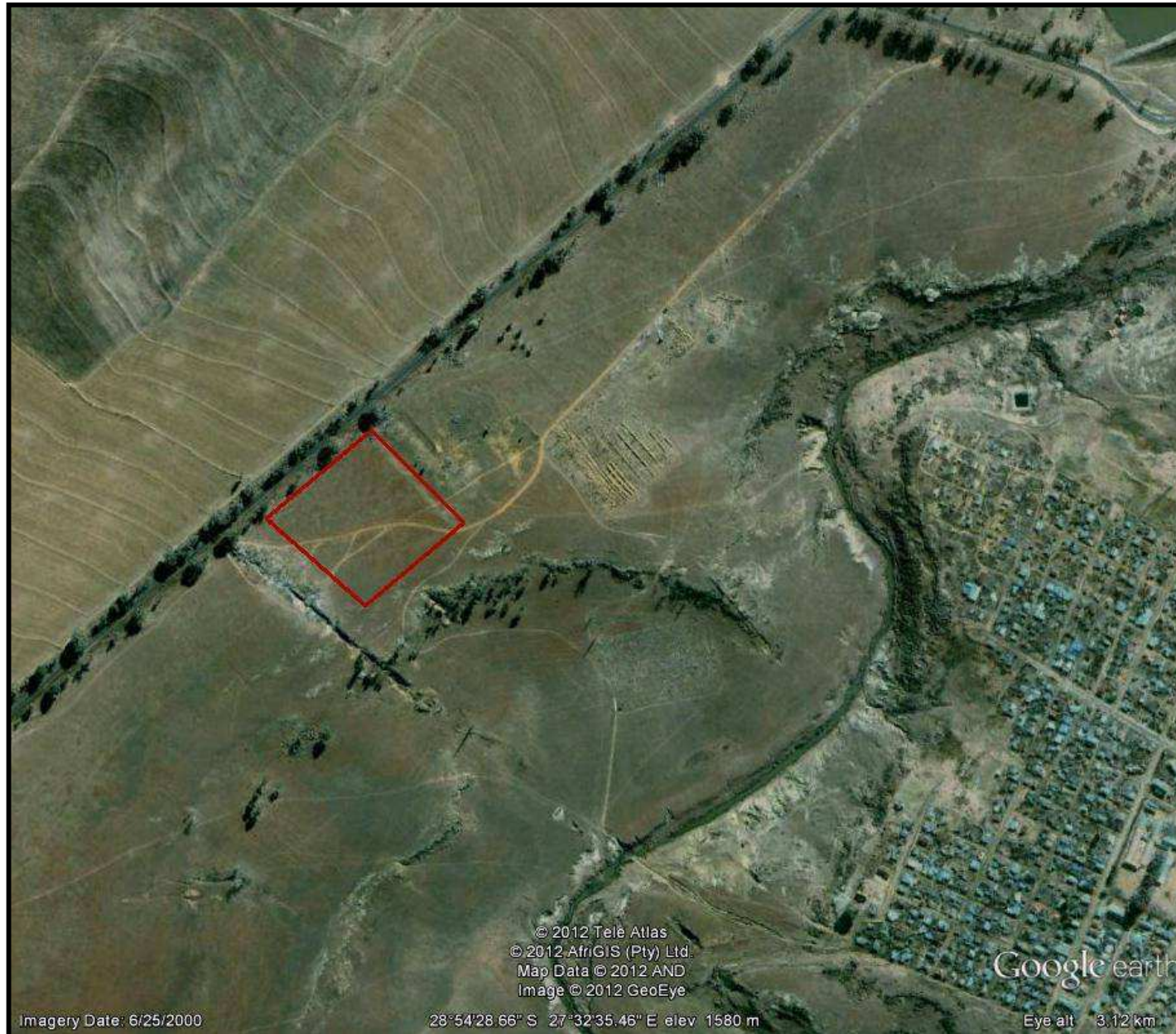
FIG. 2: AERIAL OVERVIEW OF THE CLOCOLAN SOLID WASTE SITE
