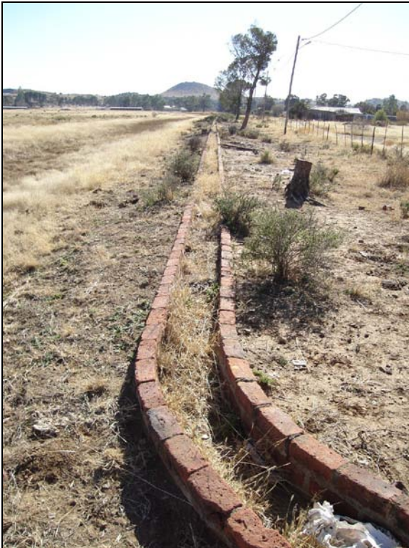
Fig.14 Irrigation furrow running into the residential area of Bethulie.
