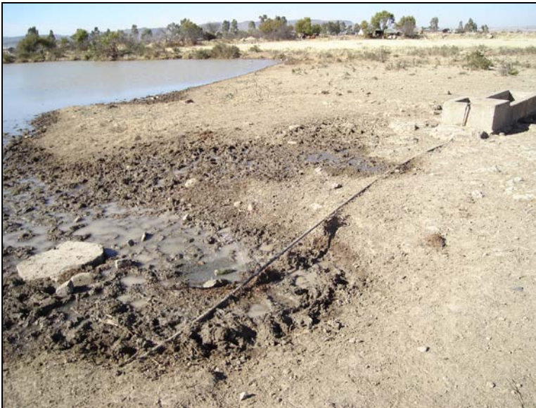
Fig.7 View of the dam where livestock come to drink.
