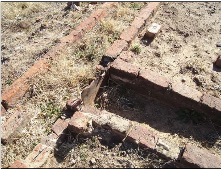
Fig.15 Irrigation water is tapped off from the mainline into the vegetable gardens.
