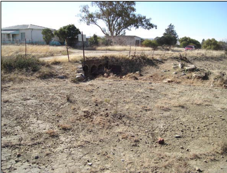
Fig.11 Storm water culvert from residential area.
