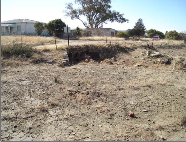
Fig.4 Culvert where storm water from town enters the proposed development area.
