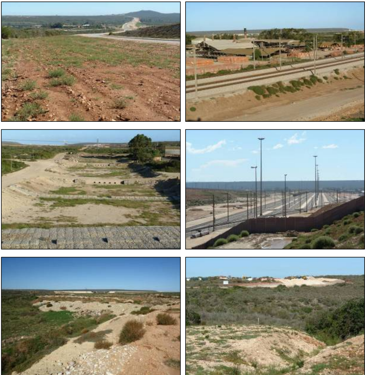
Figs 59-64. Views of the developments in Zone 9 which include brick making, the construction of roads, drainage channels, railway lines, dumping and mining activities.
