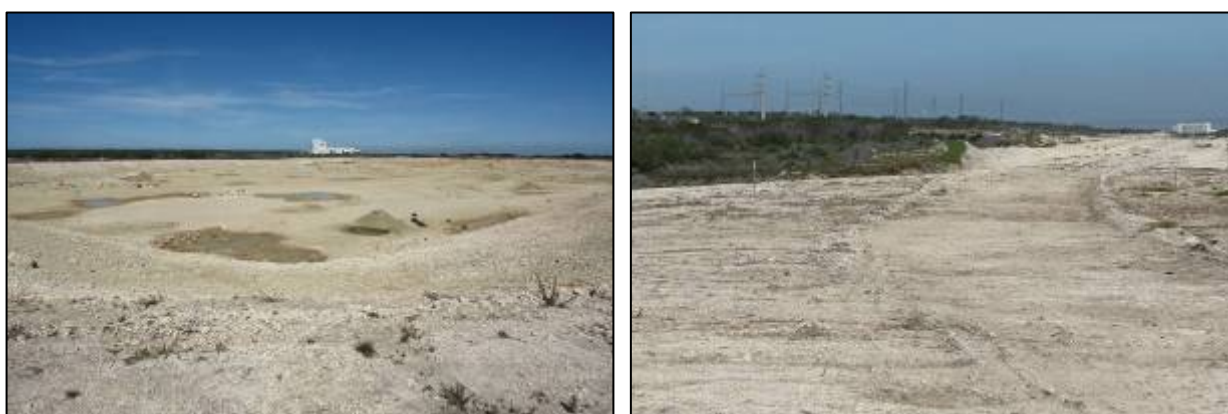
Figs 43-44. Views of the large scale damage caused recently to the landscape by quarrying, road and power sub station constructing activities in Zone 7.
