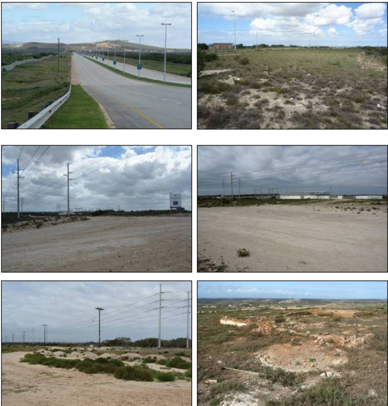
Figs 1-4. Different views of the large scale damage caused recently to the landscape by the development of the infrastructure in Zone 5.
