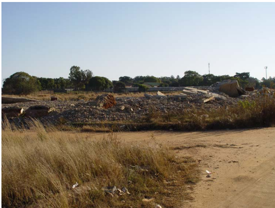
Figure 2: Large demolished structure.
