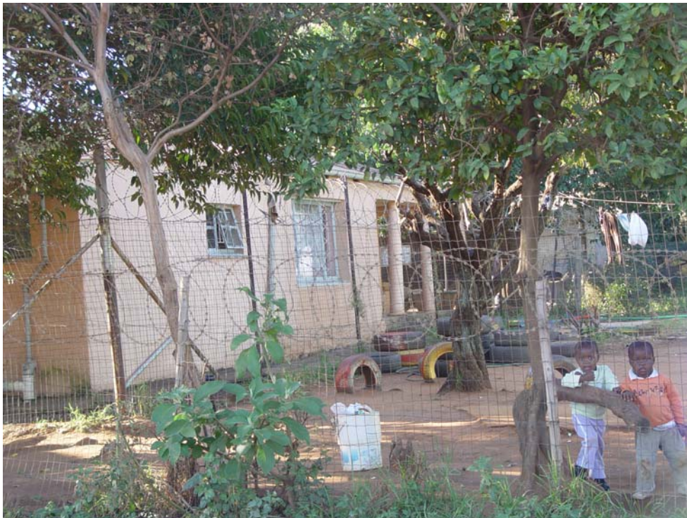
Figure 3: Multi-room brick house with corrugated iron roof.
