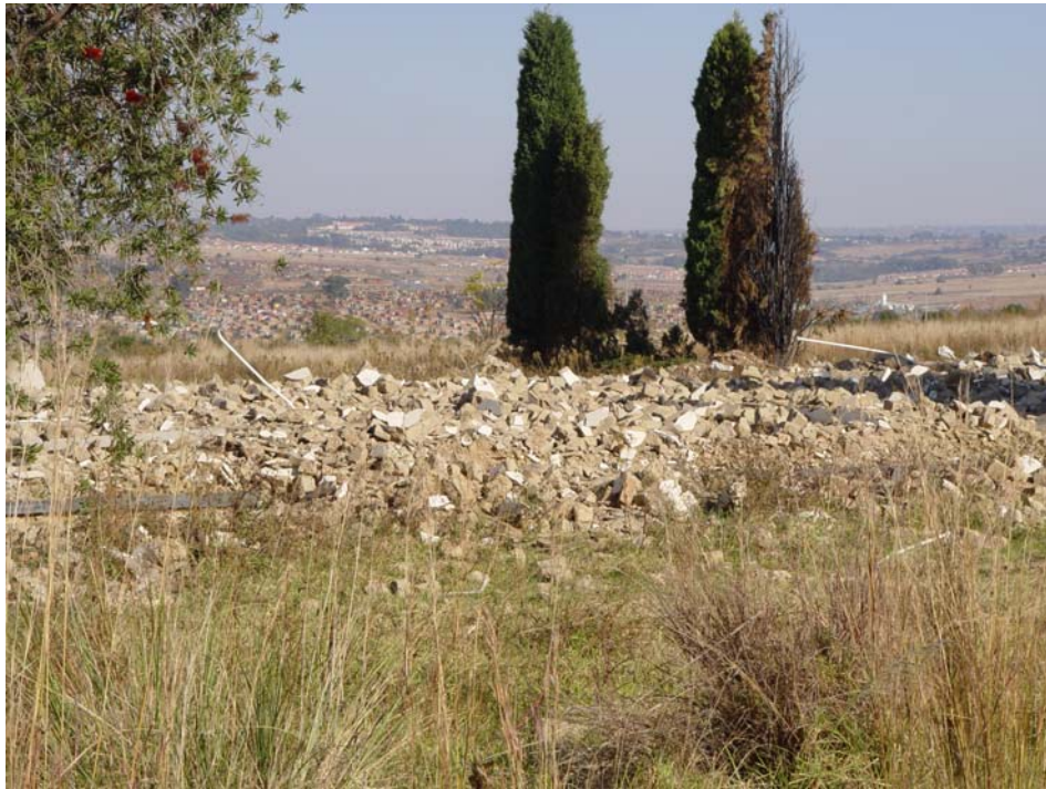
Figure 1: Demolished multi-room structure.
