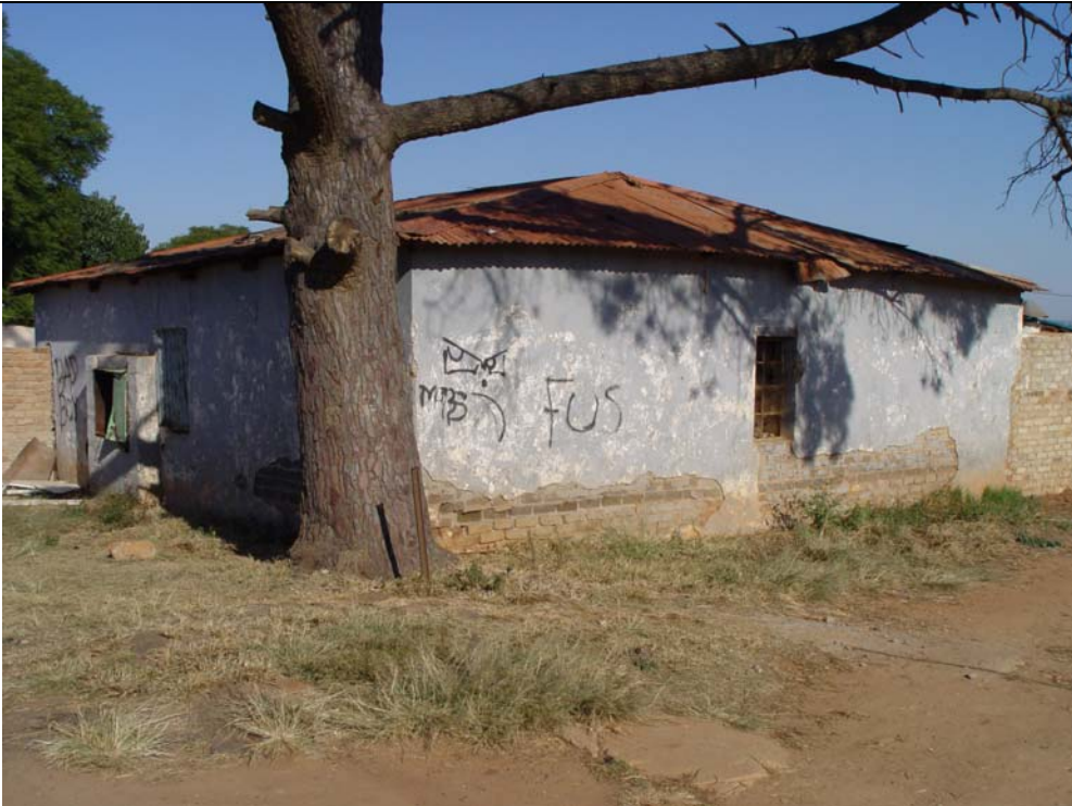
Figure 2: Multi-room brick house with corrugated iron roof.
