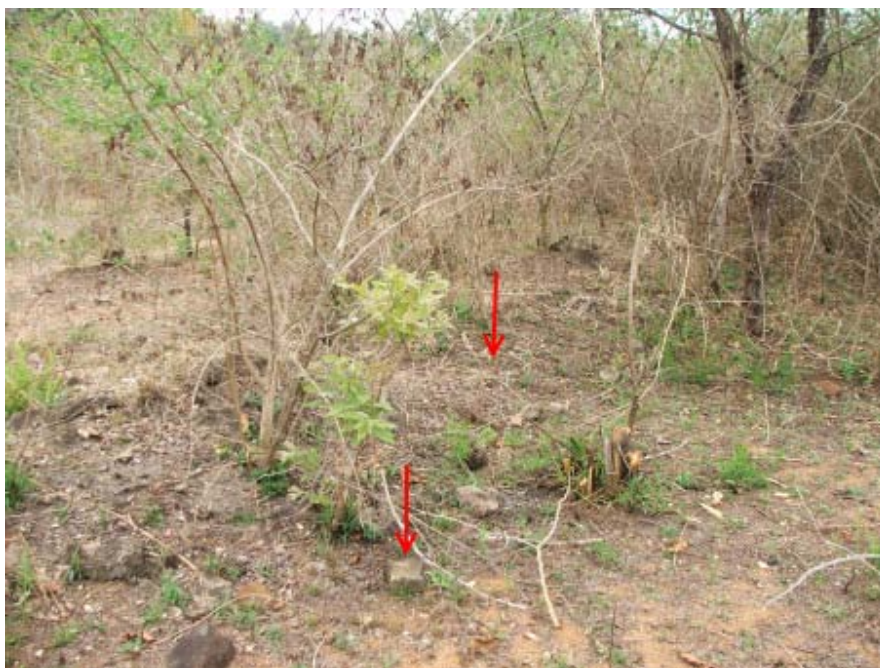
Fig. 4. Site HD 3. The remains of one of a few square structures associated with farm worker's quarters. The arrows indicate rubble and the foundations of walls.
