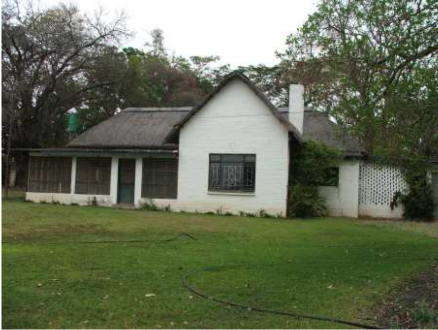
Fig. 11. Site HD 9. Main house on property. Built in 1955.
