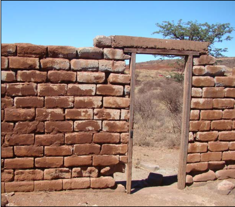
Fig.10 Wall with concrete lintel and wooden doorframe.
