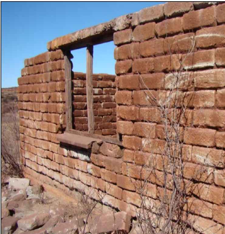
Fig.11 Wooden windowframes in the concrete walls.
