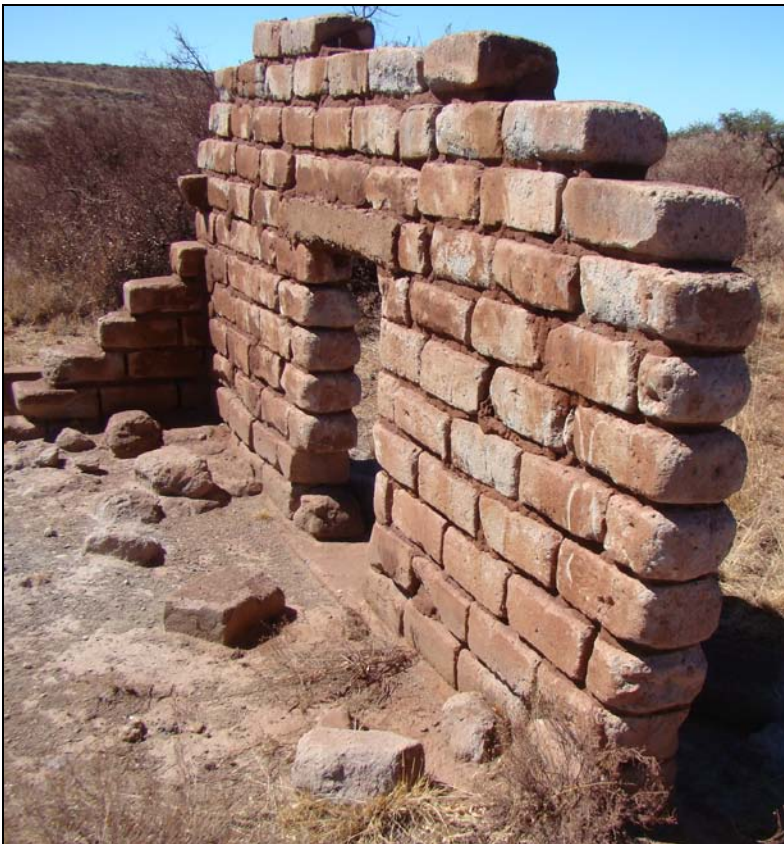
Fig.9 Wall with low concrete lintel at Demaneng.
