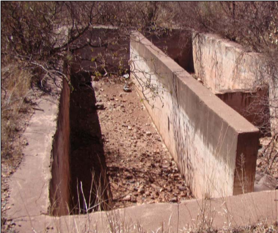
Fig.12 Concrete lined pit with dividing wall down the centre. Note water line on the wall.
