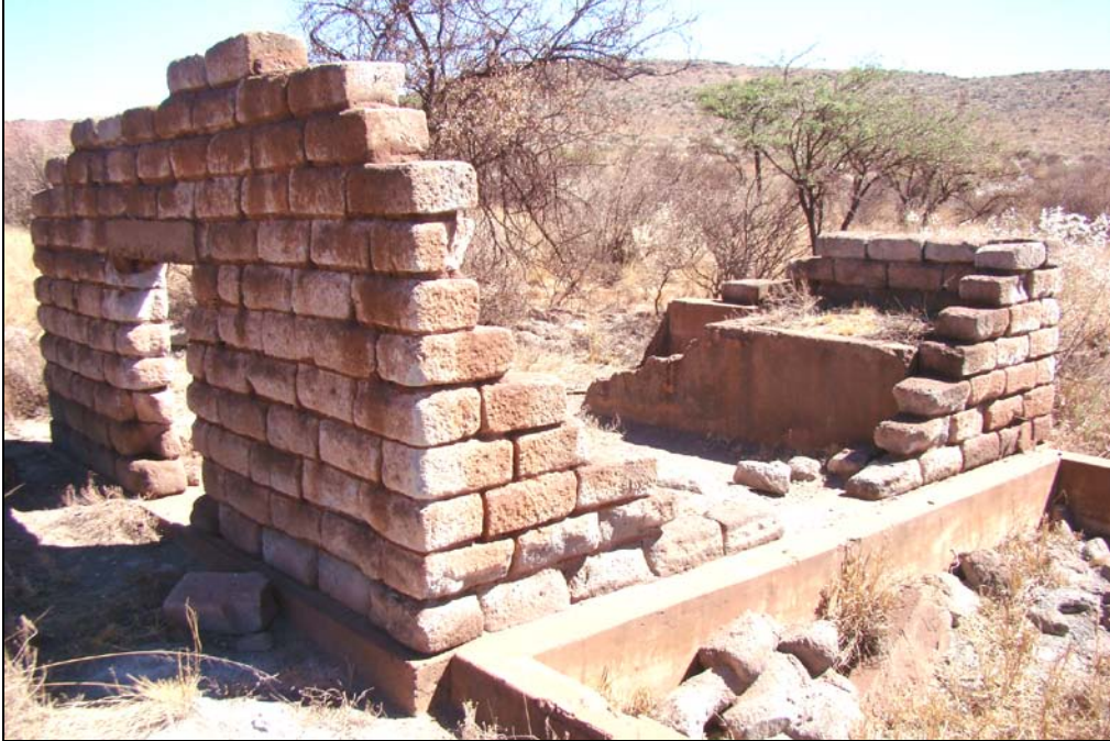
Fig.8 Ruin walls made of concrete blocks at Demaneng 546, near Kathu.
