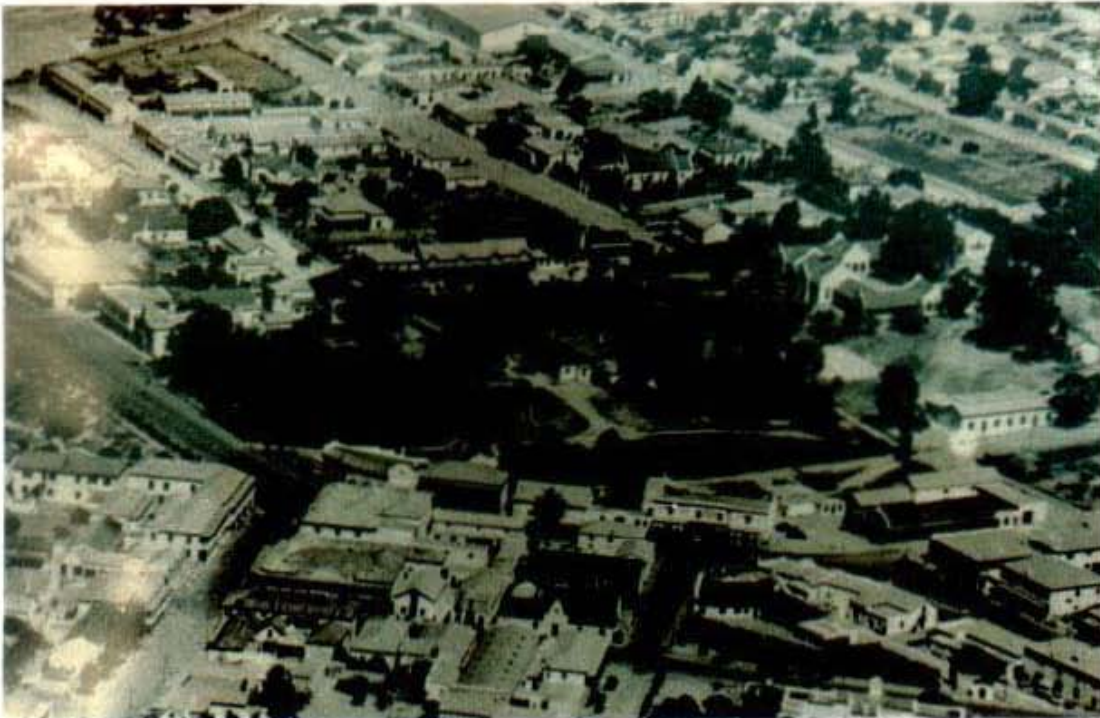
Plate 4 Aerial photograph of part of Malmesbury showing the residence and part of the baths. Copy of a framed print in the Malmesbury Museum.
