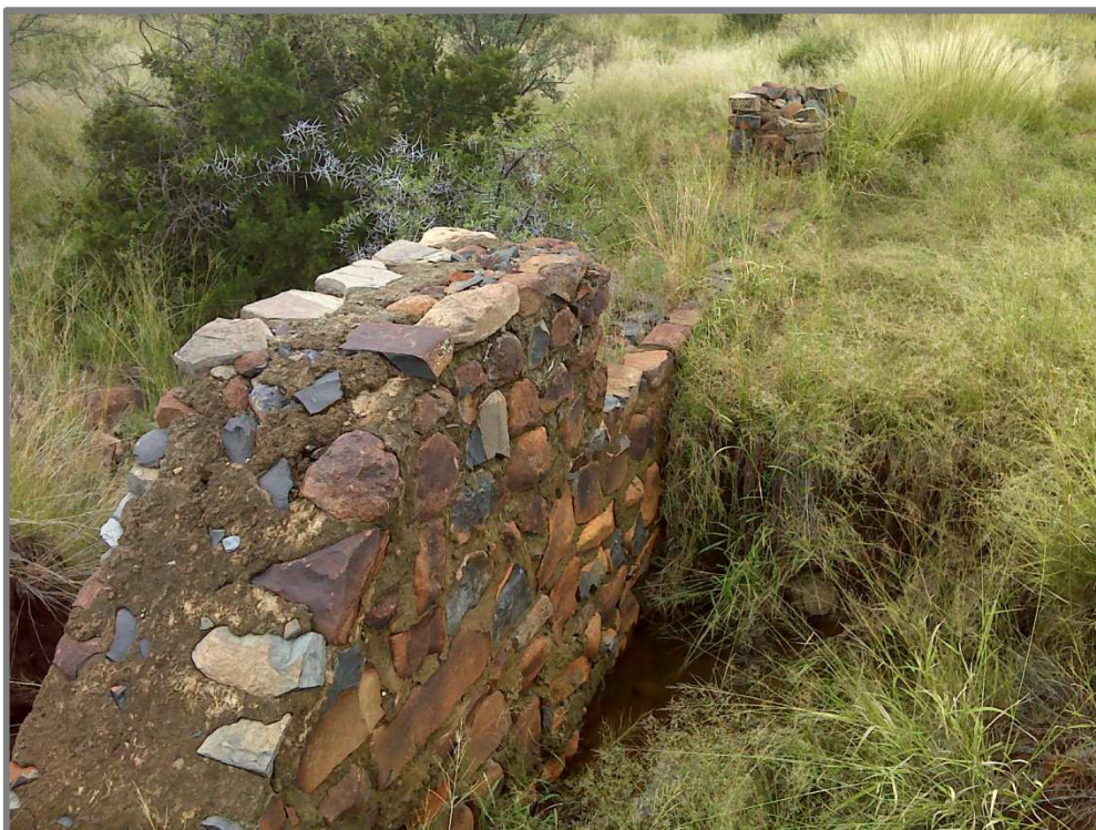
. Figure 29. Remains of the weir.
