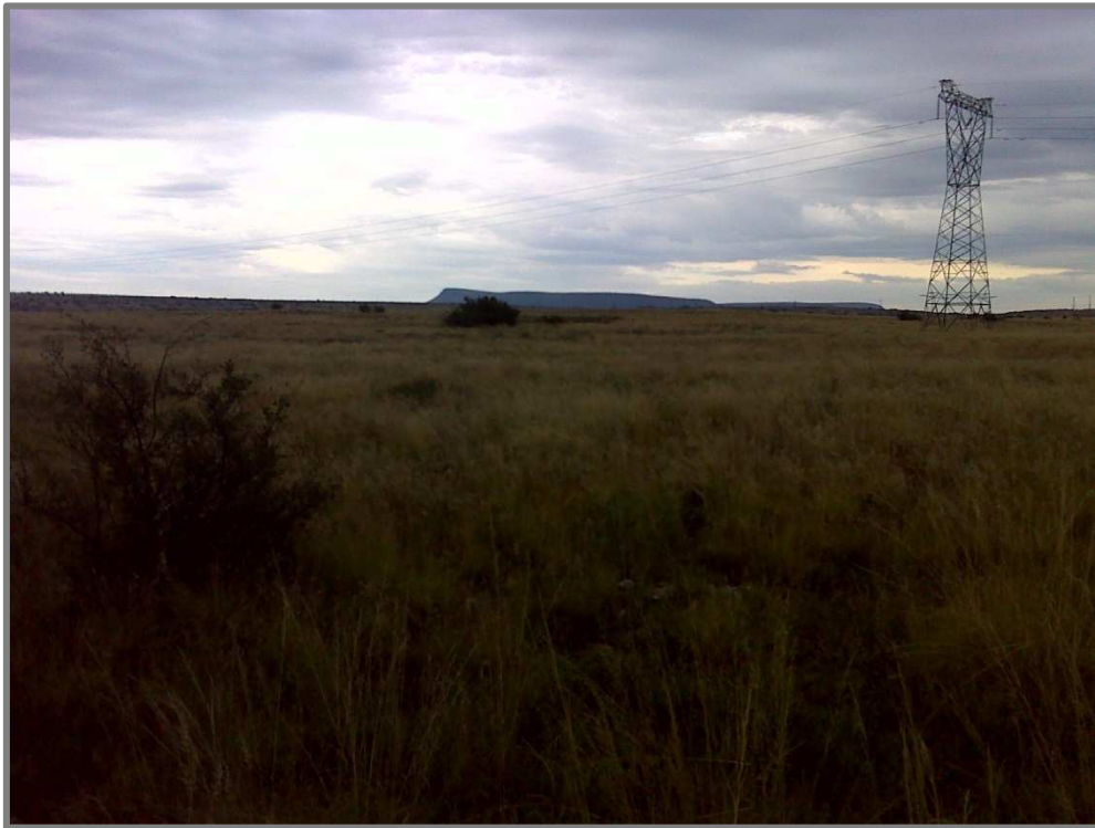
Figure 6. View of the landscape and overhead powerlines.
