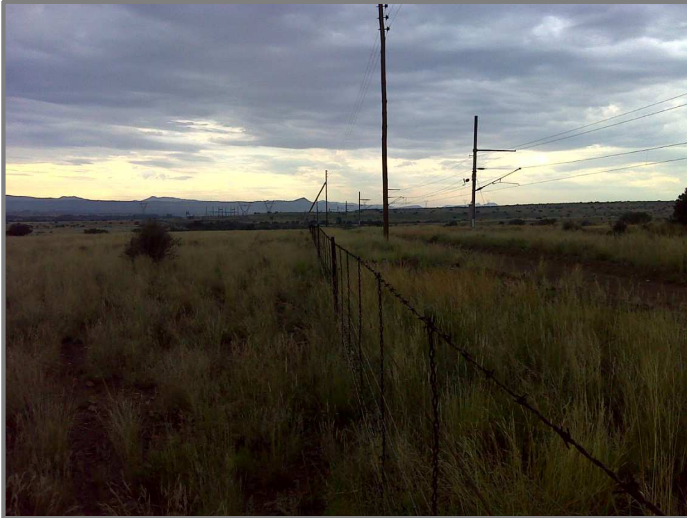
Figure 8. View of the railway facing east and the Dobbin Substation in the distance.
