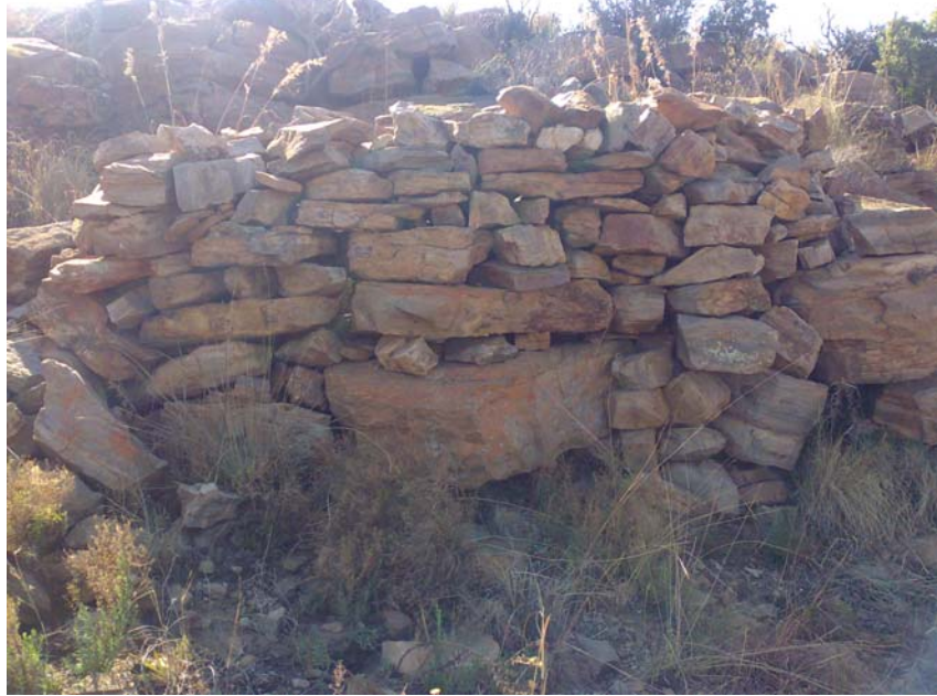
Figure 6: Frontal view of the stone walling.
