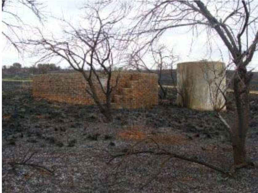
Figure 14: Site 8 – cement and brick dam
