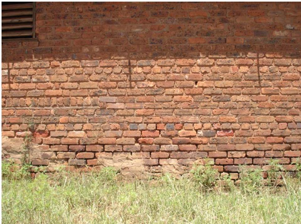
**Figure 6: English Bond building technique can be seen clearly (see row of facing bricks).**
