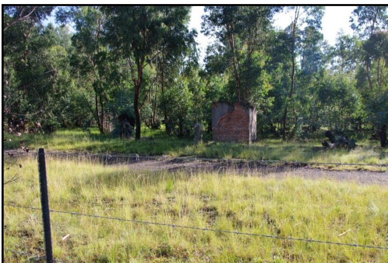
Figure 18: The outbuilding (pump station) temporarily associated with the original SITE 1 structure and located immediately adjacent to the study site
