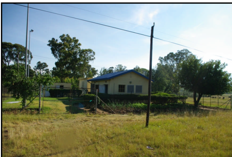
Figure 17: View of the SITE 1 structure
