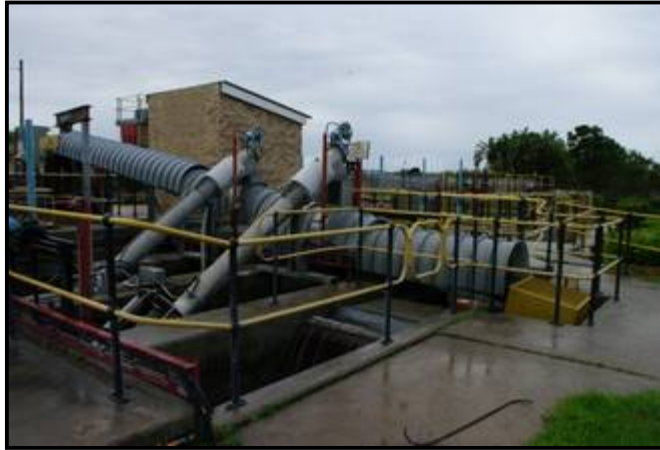
Figure 6: View of the existing Driftsands WWTW - 1
