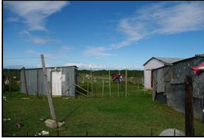
Figure 15: Existing development at the location where the line route between the Driftsands area and Walmer Township will connect
