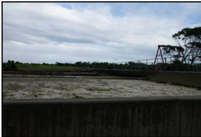
Figure 7: View of the existing Driftsands WWTW - 2
