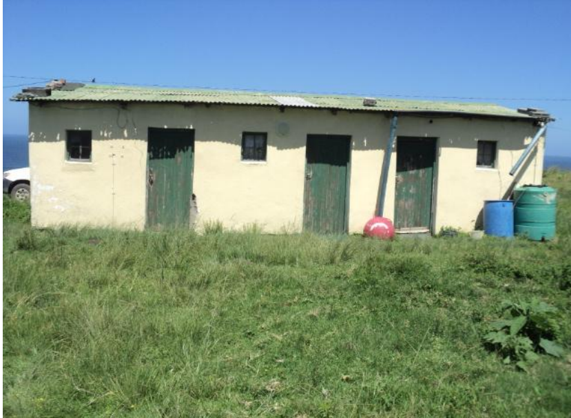
Figure 2: An overview of the three roomed structure that will be demolished.
