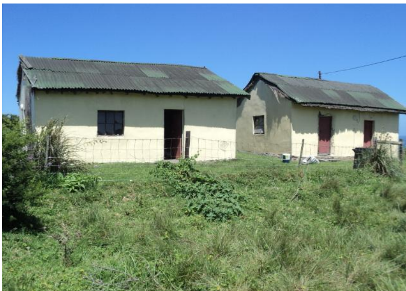
Figure 3: View of two structures that will be destroyed.
