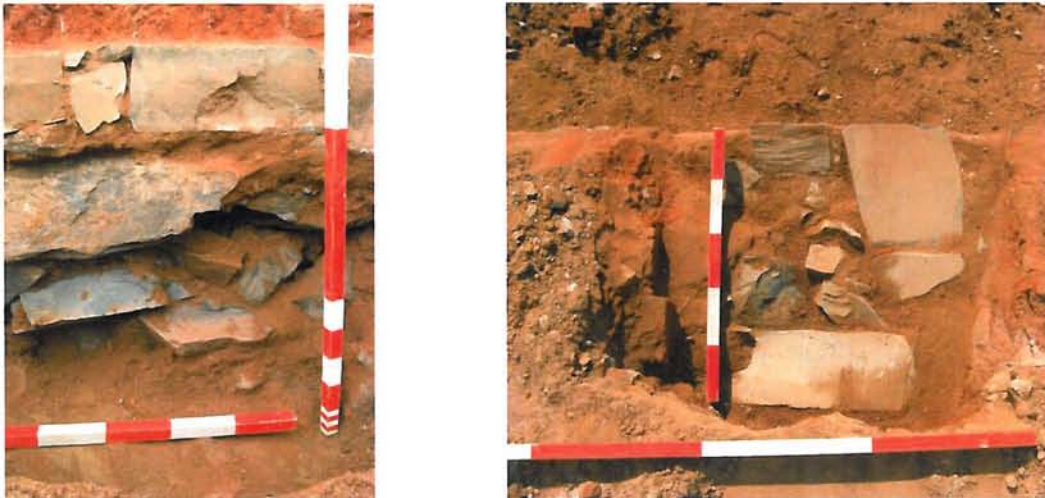
Figure 7: The foundation of the building was formed by slate rubble topped by a course of roughly dressed slate (Photograph on left). The image to the right shows the width of the walls and illustrated the construction method: roughly dressed blocks on the exterior, the interior of the wall filled by smaller chunks of rock, set in a clay/lime mortar.
