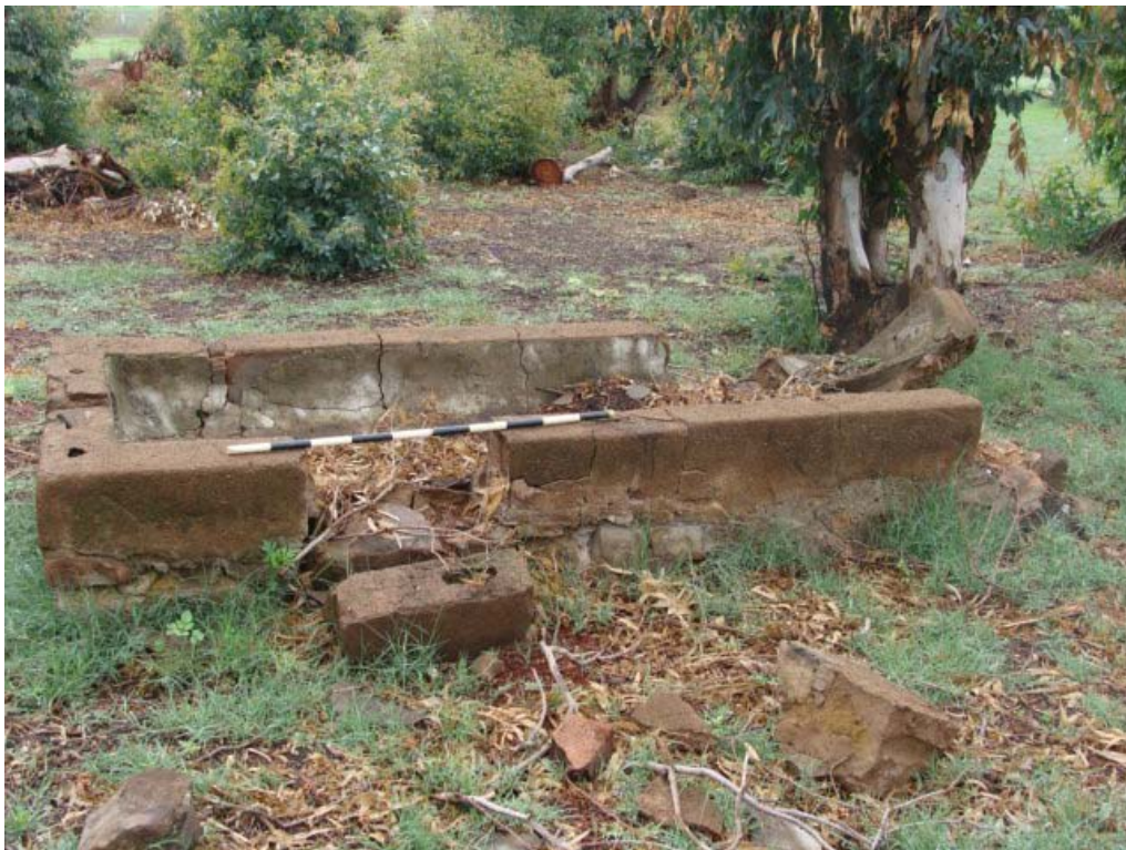
Figure 6 A water trough at site 2.
