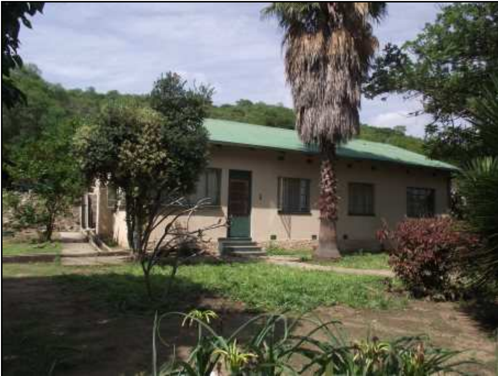
Fig. 7. Site E 4. One of the 13 houses which used to be dwellings of employees at Elandshoek Sawmill.
