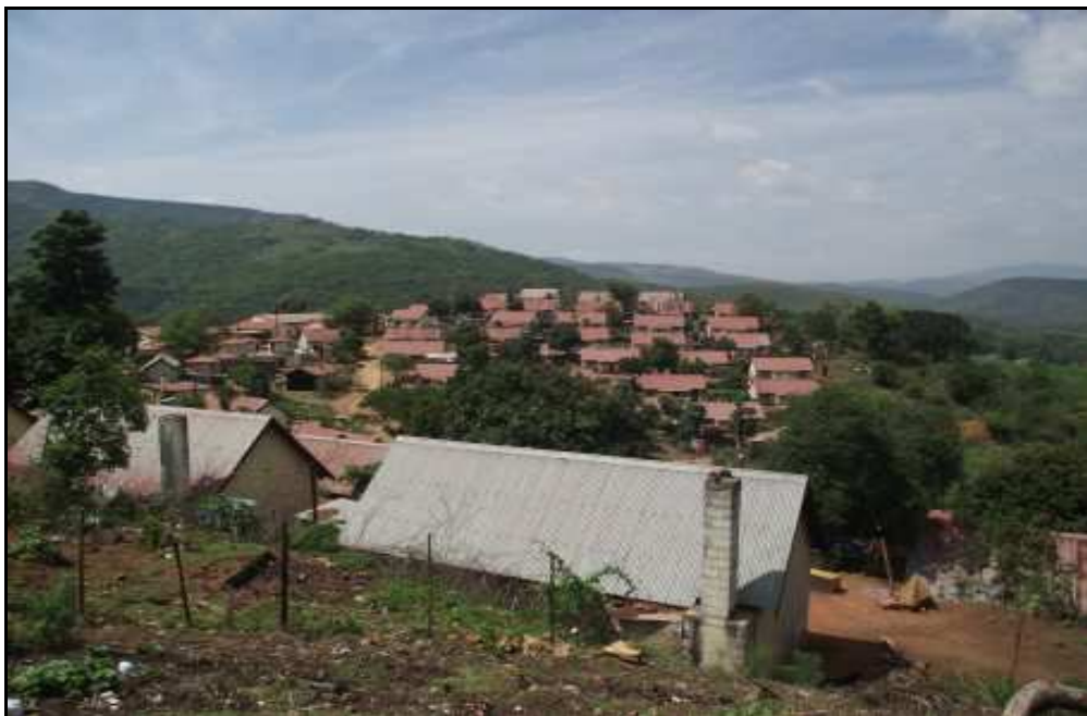
Fig. 10. Close to site E 5. Existing dwellings on the proposed development area.
