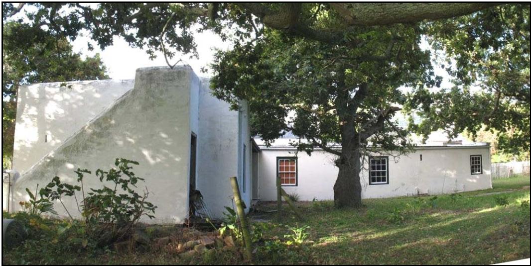
Figure 4: View of the rear of the main dwelling.
