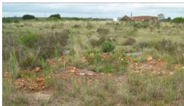
Fig.2. Some of the building rubble and buildings on the area proposed for development.
