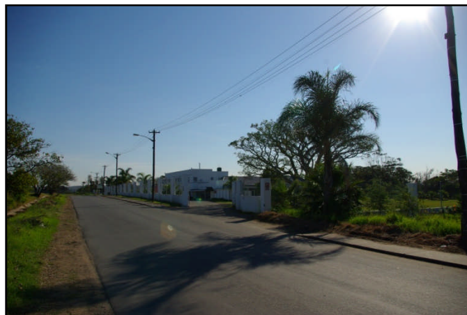
Figure 5: General view of the Orange Grove Hotel, located on Erf 49336
