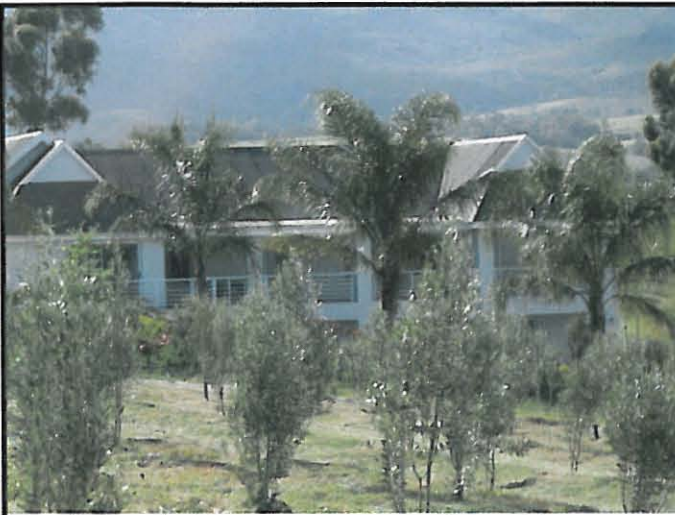
Residential house present on the central part of the site.
