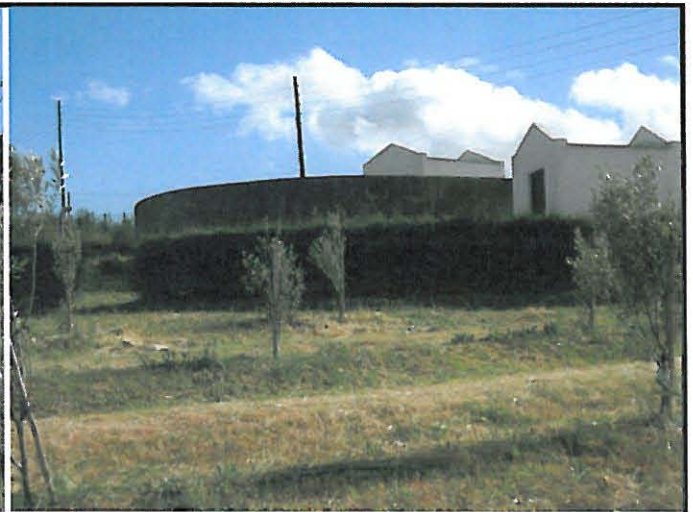
Dam present on the north-eastern corner of the site.
