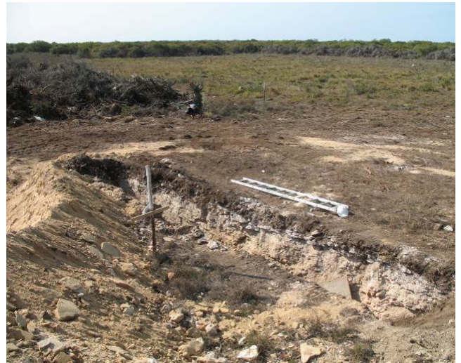
Figure 1-10: Option 1 Site. View of the site facing south east
