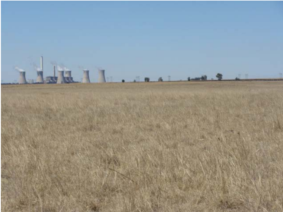
Figure 5 The Matla Power Station with natural grassland in the forefront.
