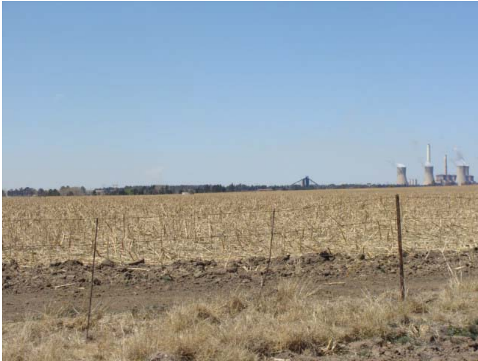
Figure 6 Maize field in the vicinity of the Matla Power Station.
