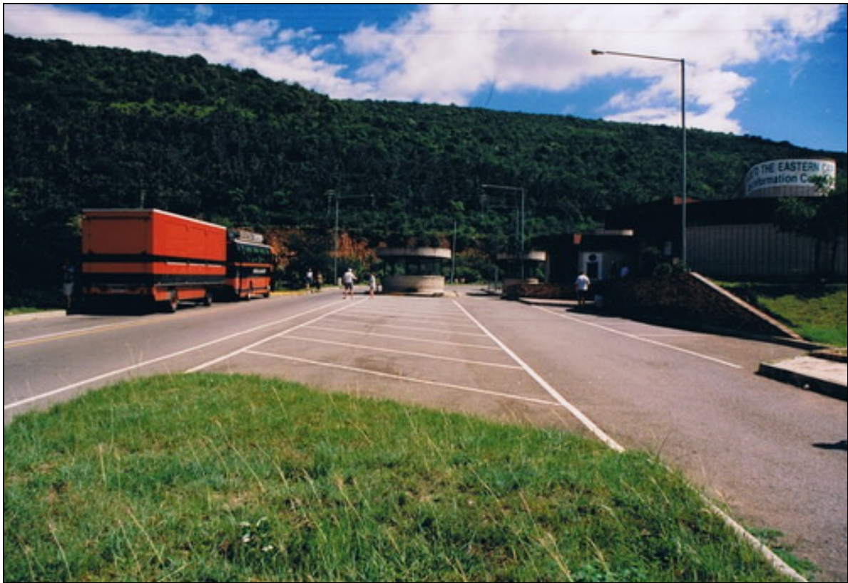
FIGURE 23: Old Transkei border post, Great Kei River Bridge
