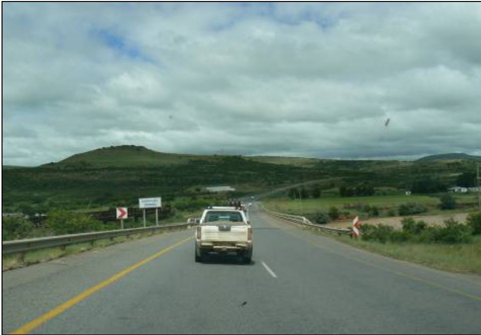
FIGURE 6: N 2 crossing the Mzimvubu River
