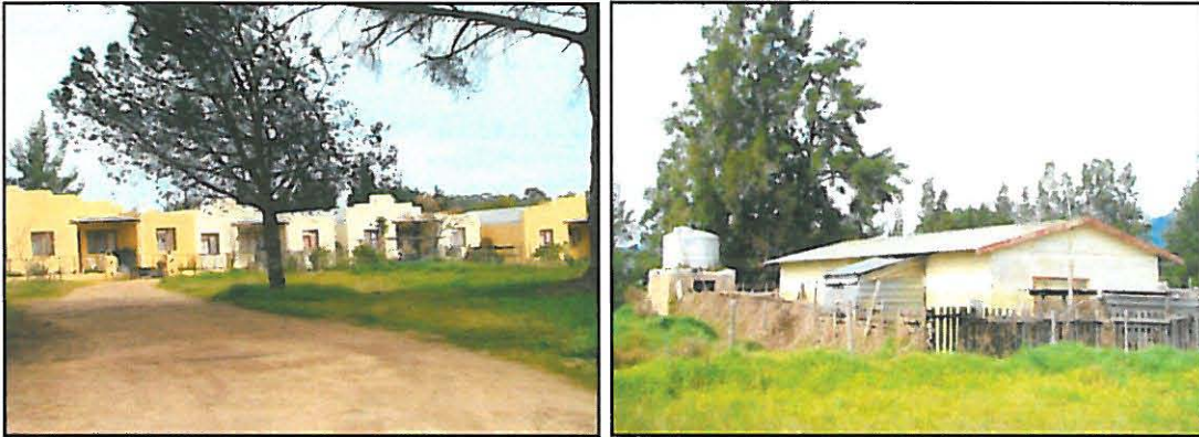
Plates 6 & 7: The housing on the property.
